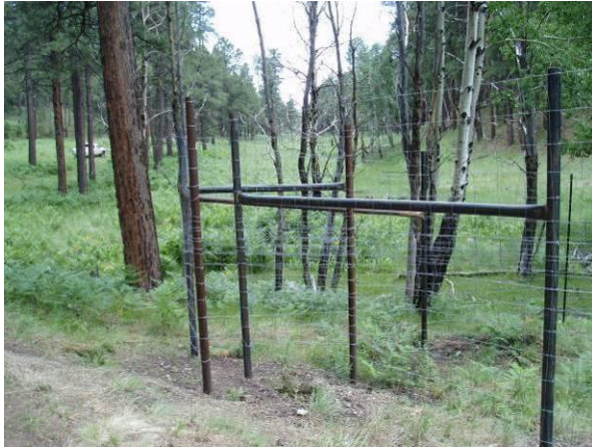
Figure 2. Example walk-through gate construction
