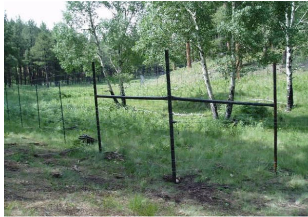
Figure 8. Example of corner construction
