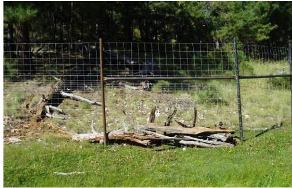
Figure 35 Large woody debris placed along bottom of fence, September 2008.
