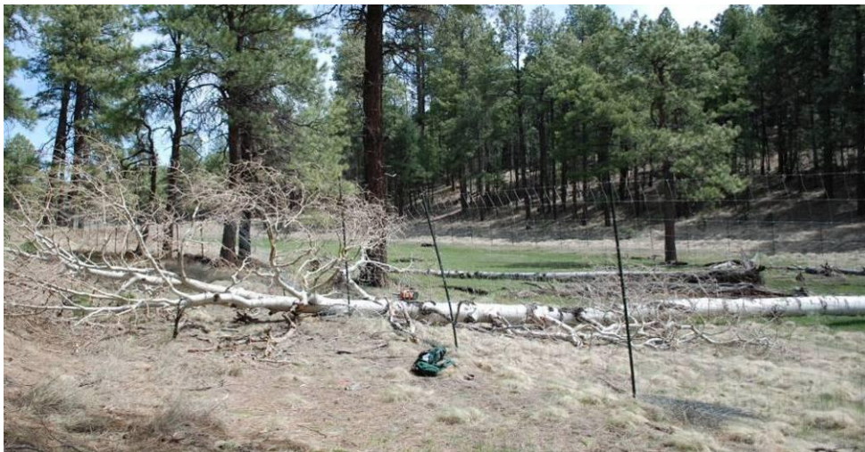
Figure 30. Fence damage from aspen, May 9, 2010.
