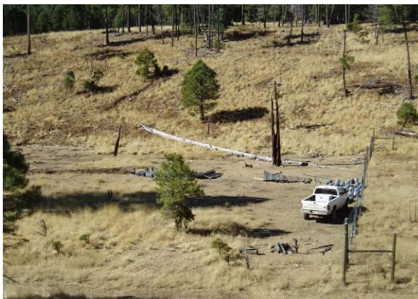
Figure 9. Fence material staging area
