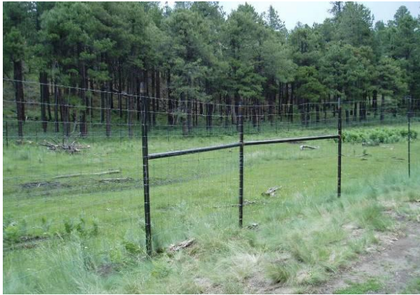
Figure 7. Example double H brace construction
