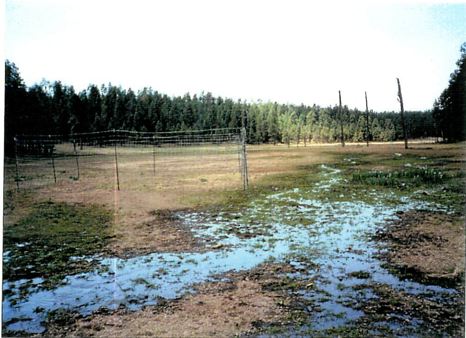
A newly constructed exclosure to monitor vegetation growth in the Gooseberry Watershed
