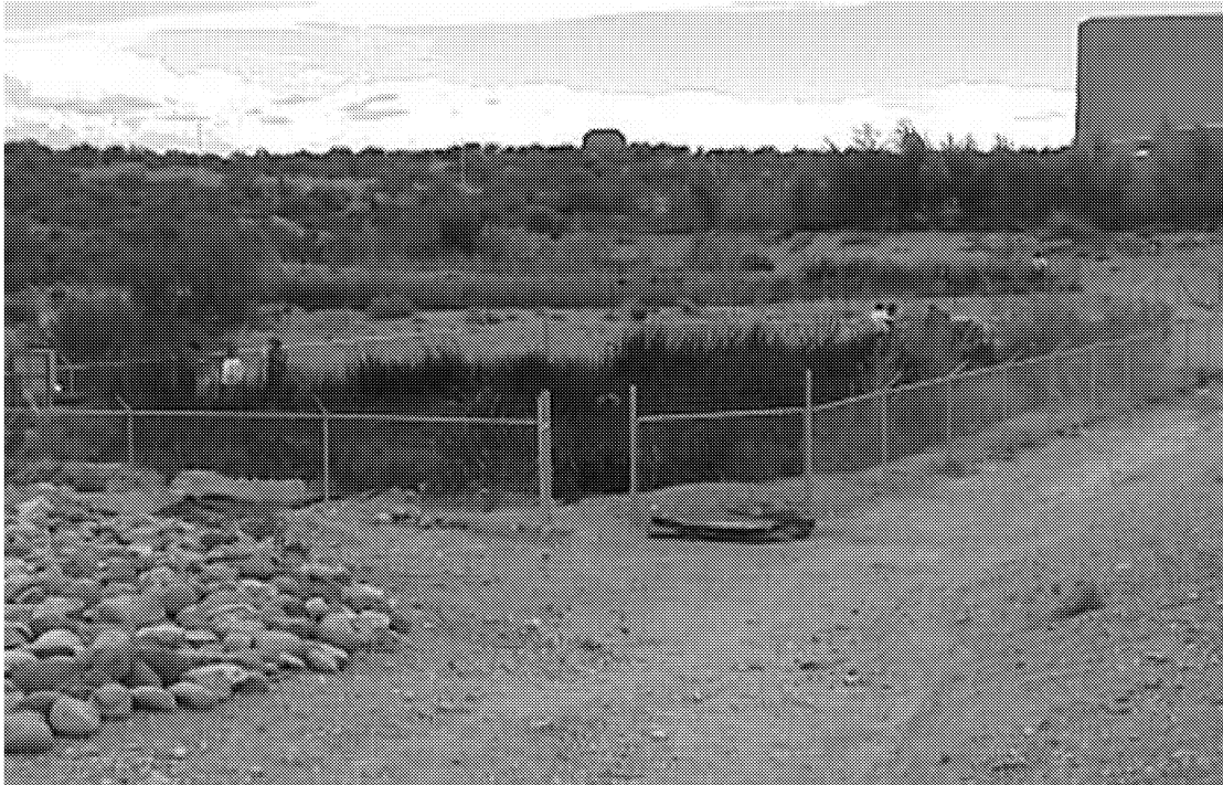
Figure 21. Portion of the wetland facility at Wickenburg High School. 99-088WPF
