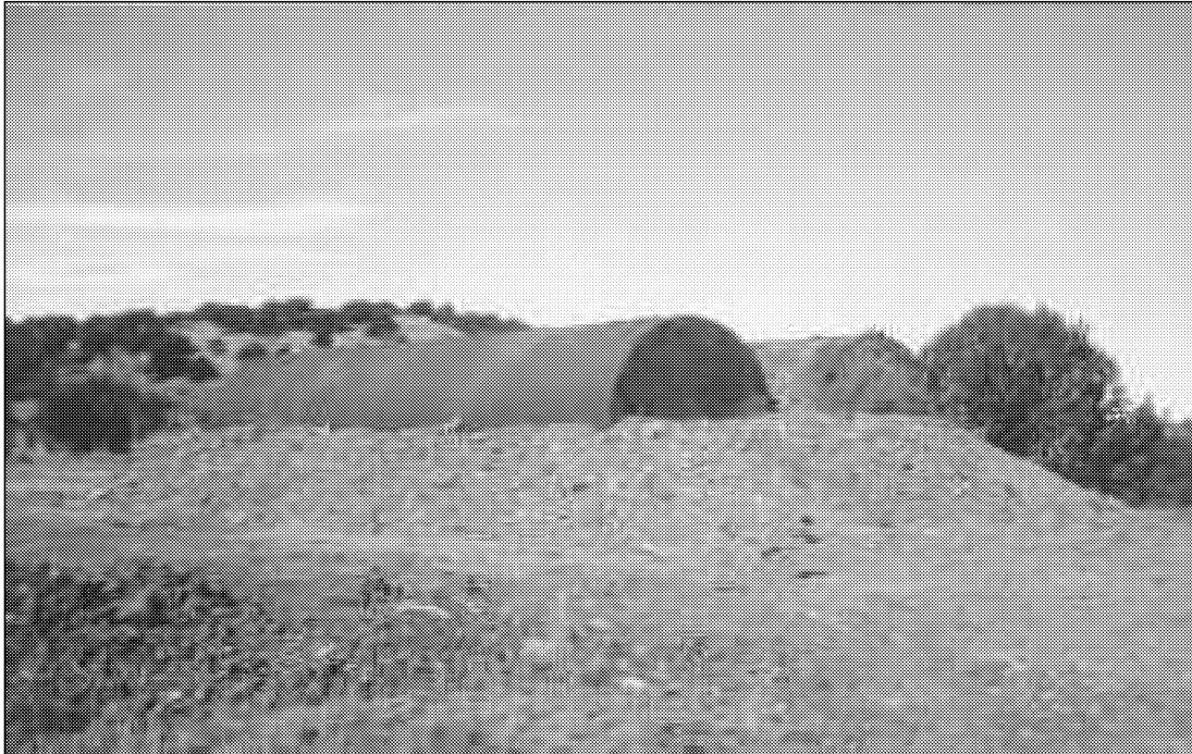
Figure 16. Two 20,000 gallon storage tanks to provide water replacement facilities upland. 98-047WPF
