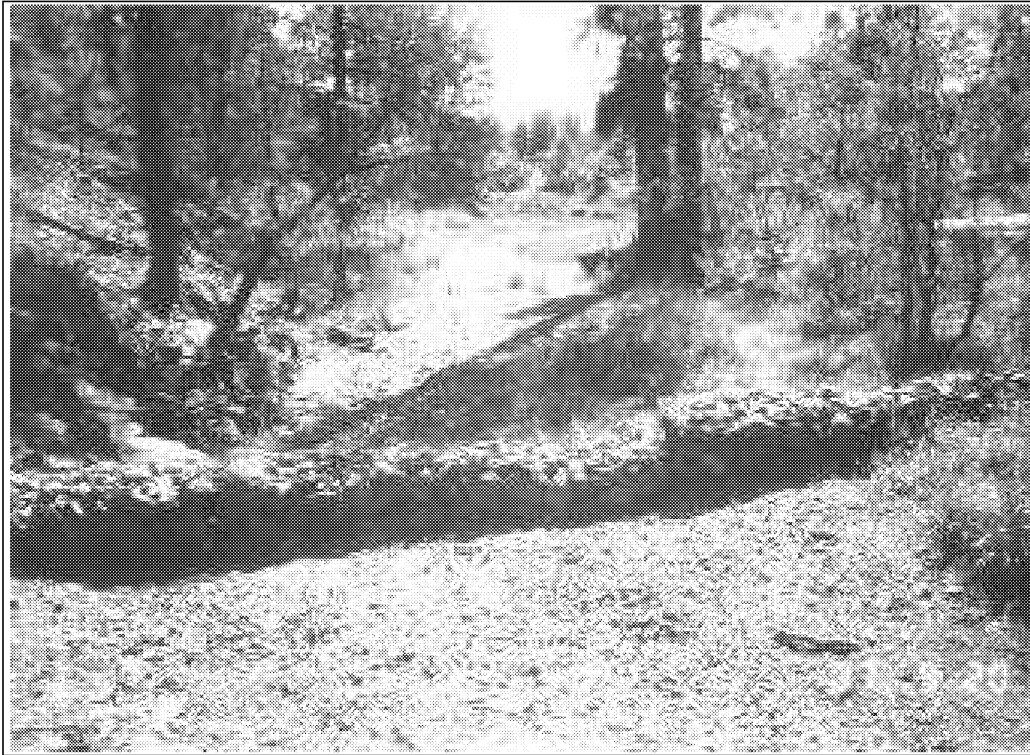
Figure 8. Erosion Control Structure at Mingus Springs Camp. 96-007WPF
