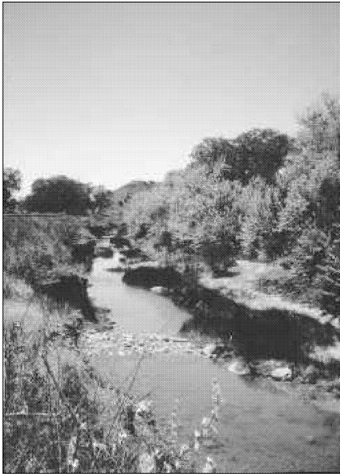
Figure 14. Low-tech in-stream structures were installed to restore meanders and pools along a portion of the Pueblo Colorado Wash at the Hubbell Trading Post National Historic Site. 97-029WPF.
