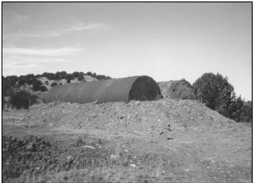
Figure 16. Two 20,000-gallon storage tanks to provide water replacement facilities upland. 98-047WPF
