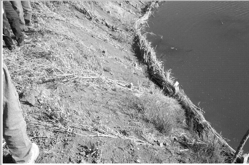
Figure 23. The Little Colorado River Enhancement Demonstration Project is using natural channel design approaches to restore a segment of the Little Colorado River. 99-092WPF
