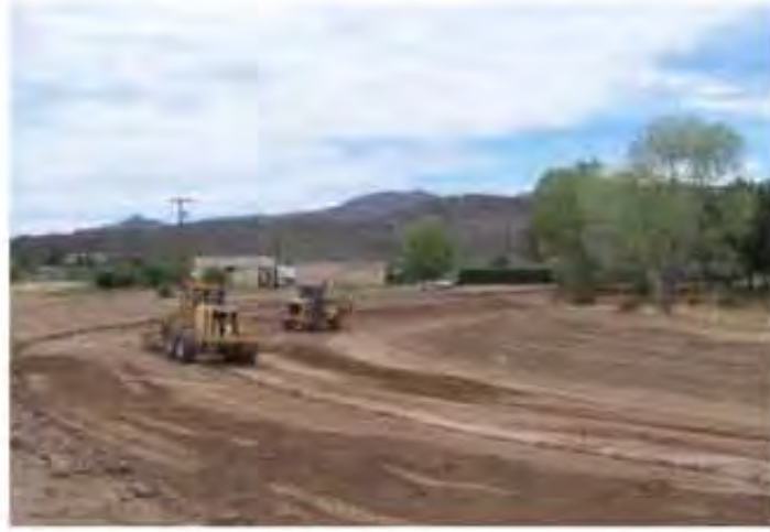
Recontouring of the existing the ponds
