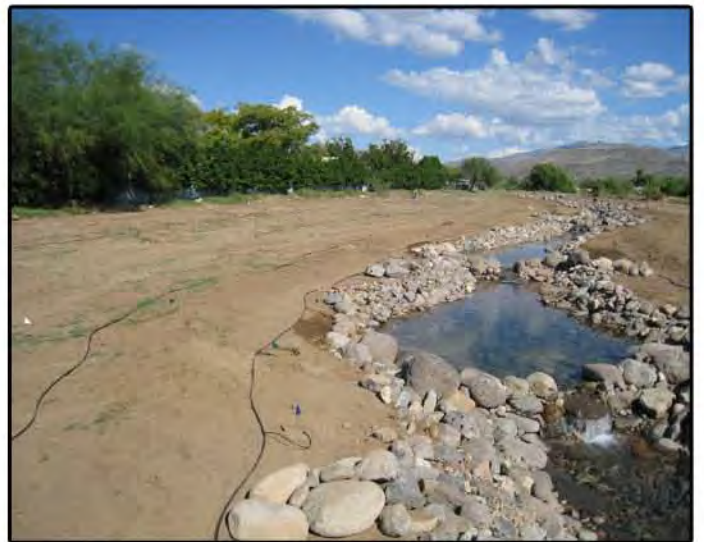
Irrigation lines next to stream & pools
