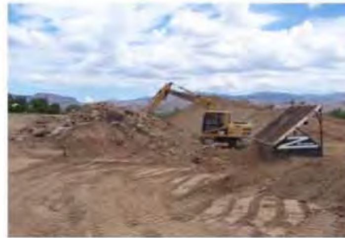
Screening excavated native material
