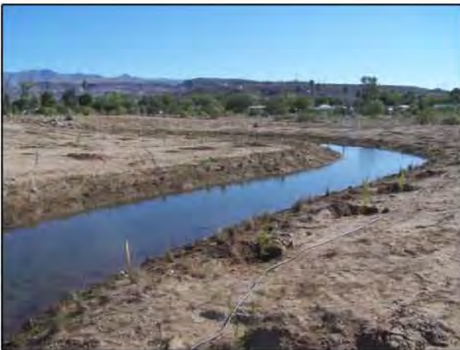
Wetland channel after planting
