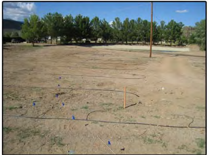
Irrigation lateral lines at the entrance to water grass meadow
