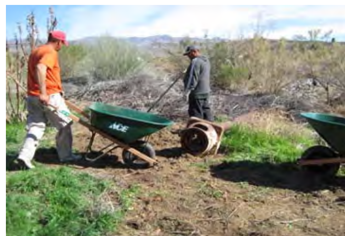
Clean up of the old mulch pile.
