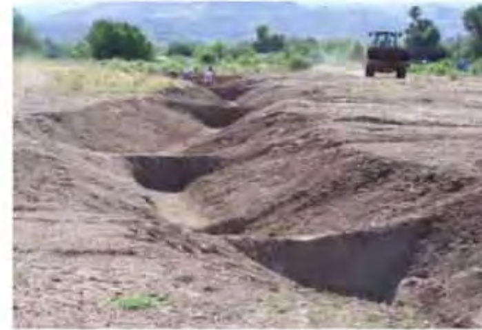
Construction of the stream and wetland channel
