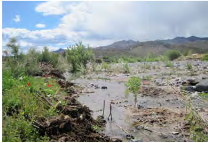
Vertical bundles staked into bank line approximately 150 yards upstream of bridge.
