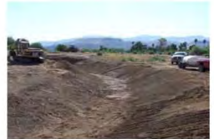
Construction of the stream and wetland channel
