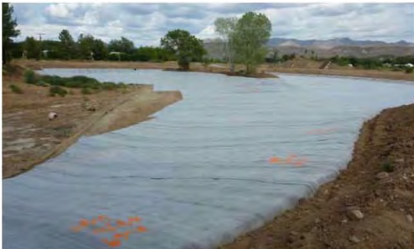
Liner covering the re-contoured pond area
