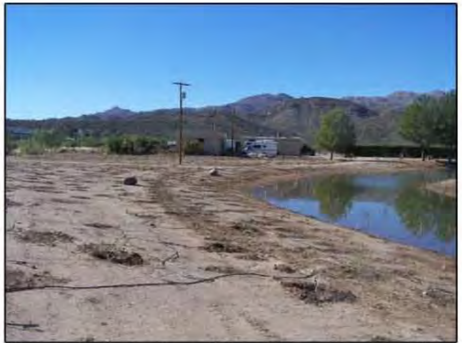
Completed planting of riparian zone around the wetland/pond
