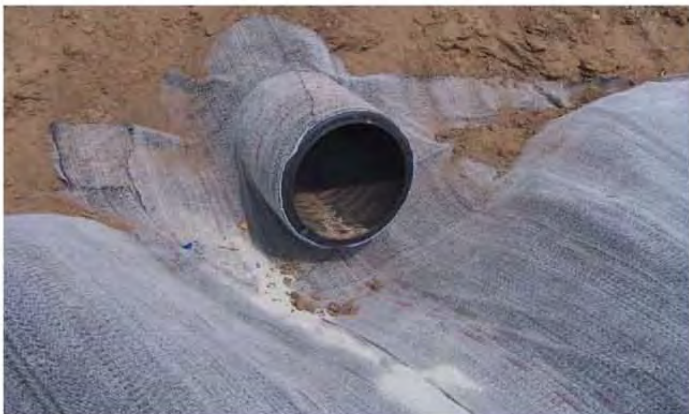
Outfall of the stop log structure
