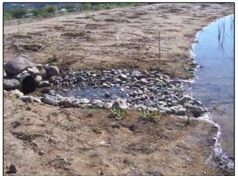
Completed plantings around the outfall of the stoplog structure
