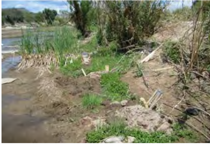
Vertical bundles staked into bank line approximately 150 yards upstream of bridge.
