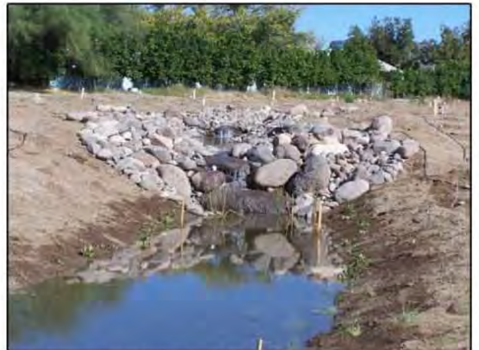
Completed wetland channel and waterfall
