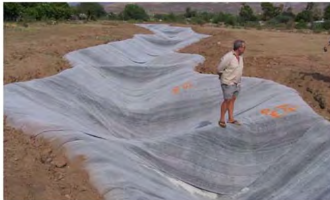
Liner covering the stream and pool system
