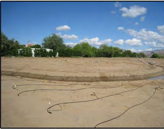
Irrigation PVC lateral lines and emitters next to wetland channel to water cottonwood/willow habitat
