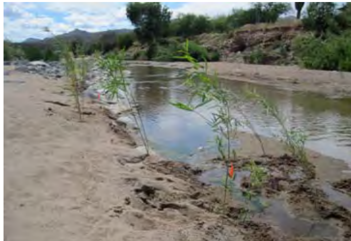
Sandbars with 1 gallon willow plantings at upstream terminus of project.
