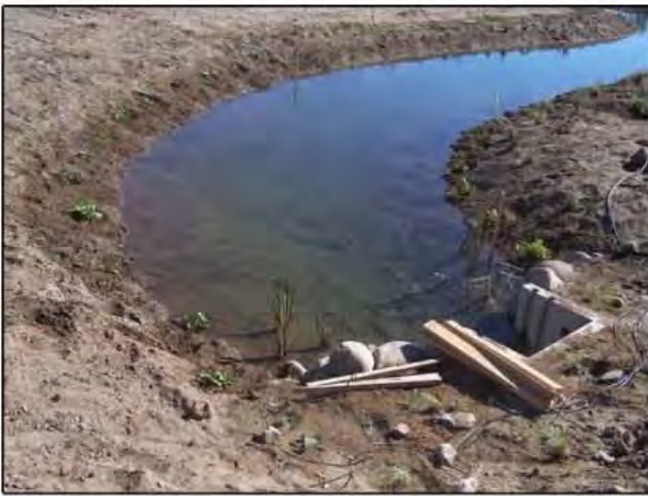
Completed plantings around the stoplog structure
