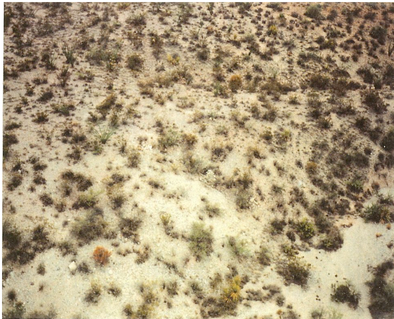
Aerial photo of check dam structures in a tributary in Teran Watershed in 1997 just after construction.
