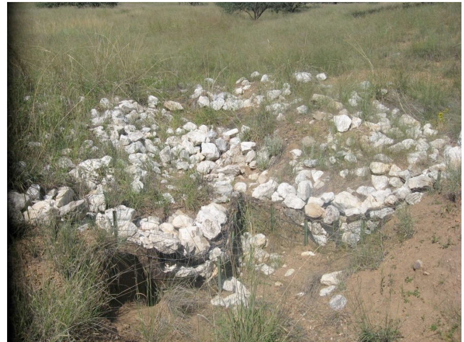
Low rock structures were installed to stabilize headcutting. September 2007 .
