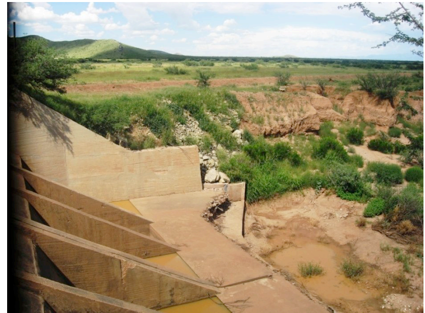
Spillway five years after project completion. August 2007.
