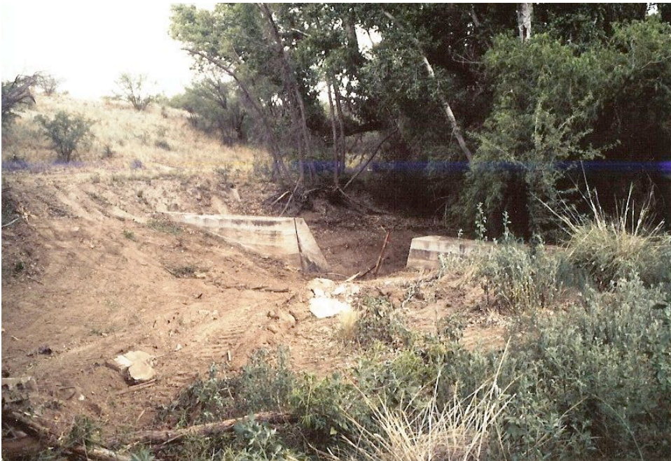
Stream channel prior to the removal of Dam #2 to be removed.
