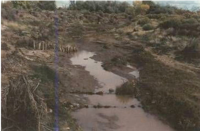
Post vane installation, November 2000.
