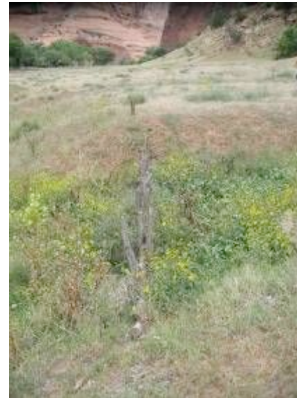
Erosion fence with sediment filled behind, Demo Site #5, October 2007.
