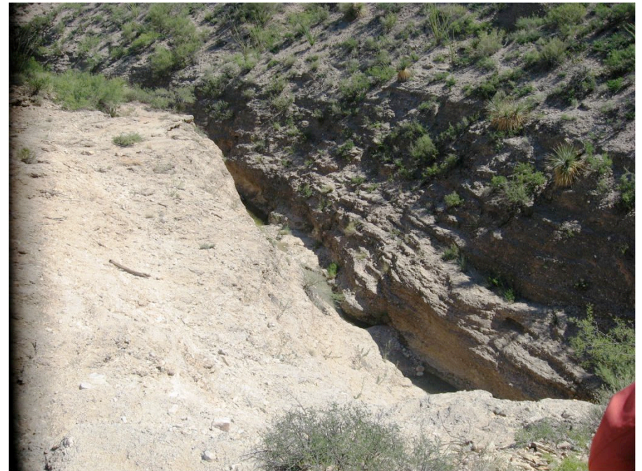
Drainage channel that stock tank leaks into. August 2007.
