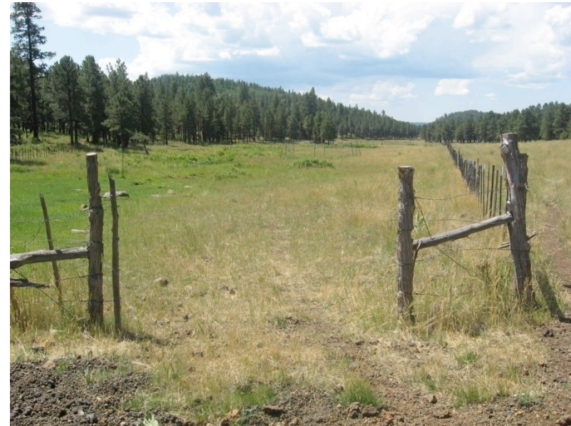
Fences are intact, however gates are open allowing livestock access to sensitive areas.
