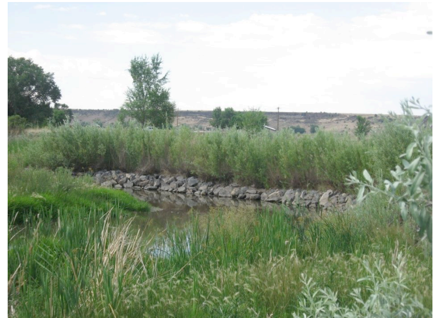
Toe rock and willow plantings used to stabilize banks on the Little Colorado River Demonstration Project.
