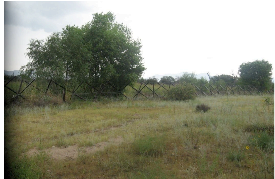
Native riparian species were planted along the stream bank behind the Kellner Jacks for erosion protection and habitat. 2007.
