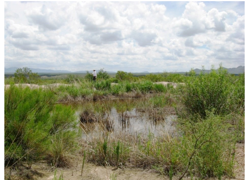
San Pedro Riparian National Conservation Area . Berm created during 95-015 to trap water and stop advancing headcut on the downstream side. July 2007.
