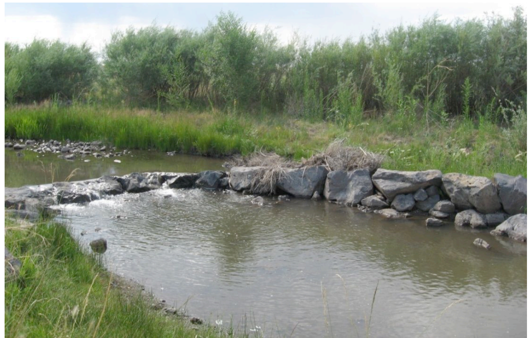
Rock weir installed for grade control and water diversion demonstration.
