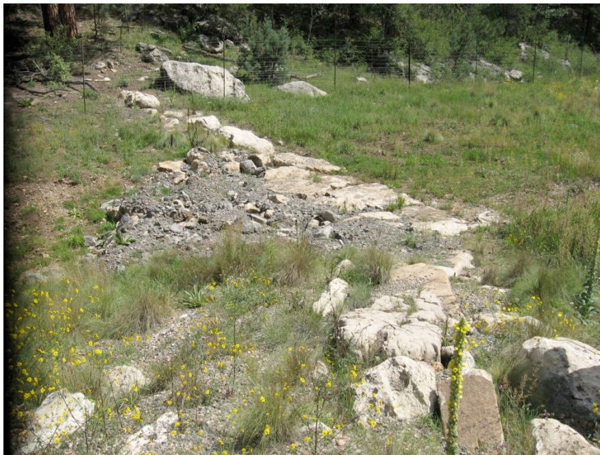
Large drop structure at downstream end of project. September 2007.
