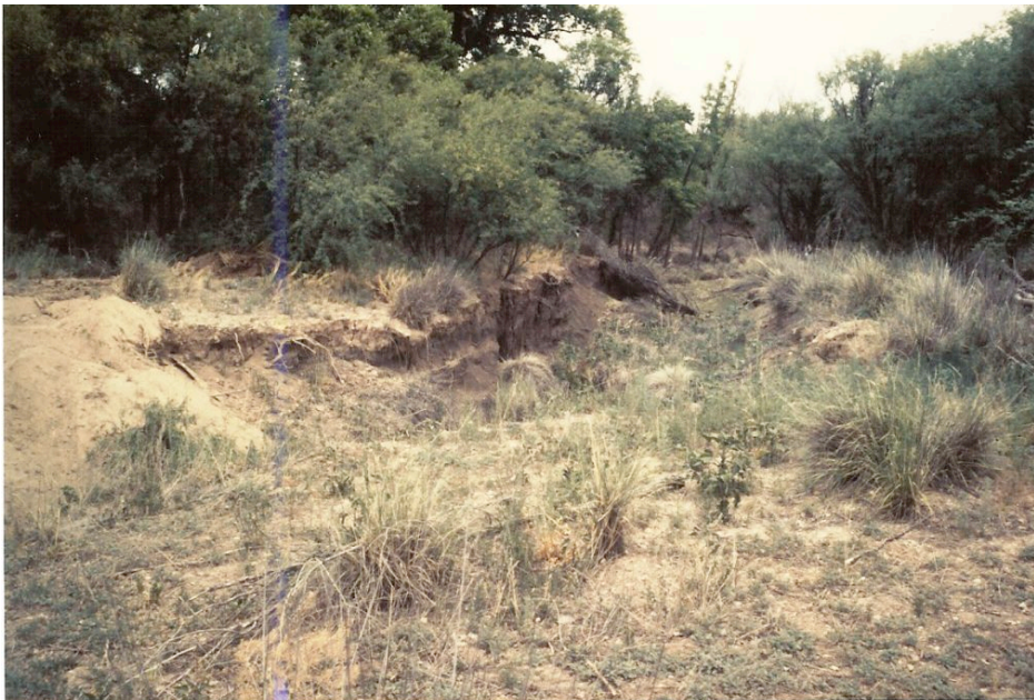
Downstream view of the advancing headcut below Dike #3 prior to implementation of grant tasks.
