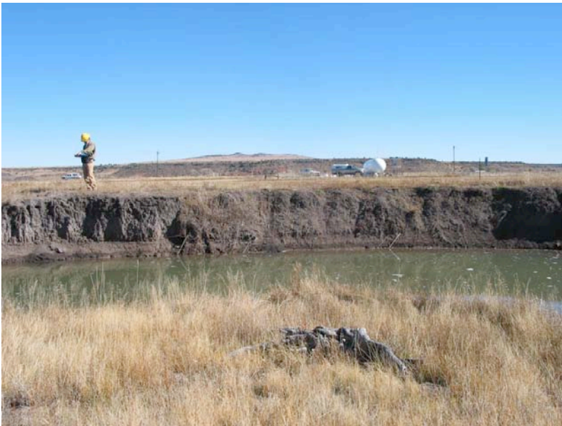
Typical eroded bank along Little Colorado River in 2002.
