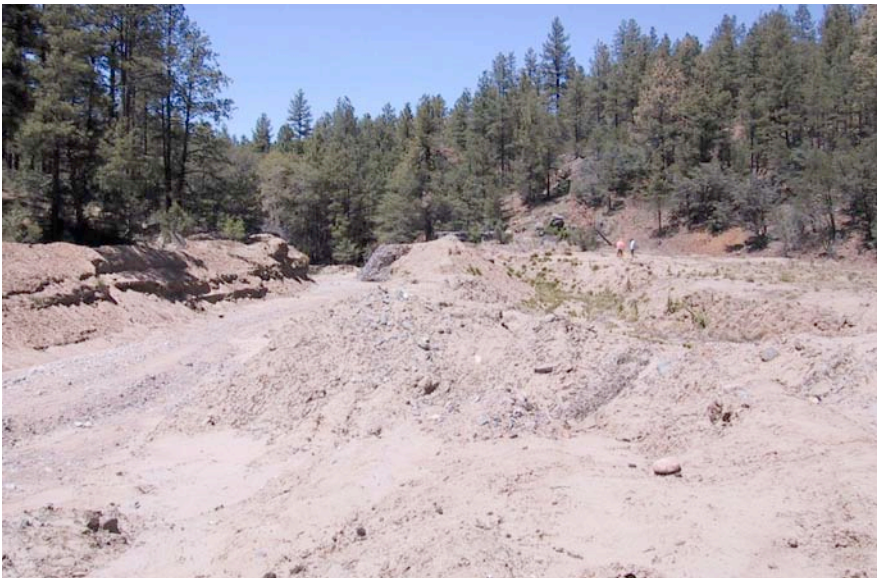
Sediment accumulation upstream of gabion dam. September 2003.
