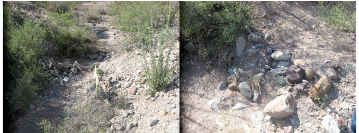
Check dam remnants on remaining structures in 2007
