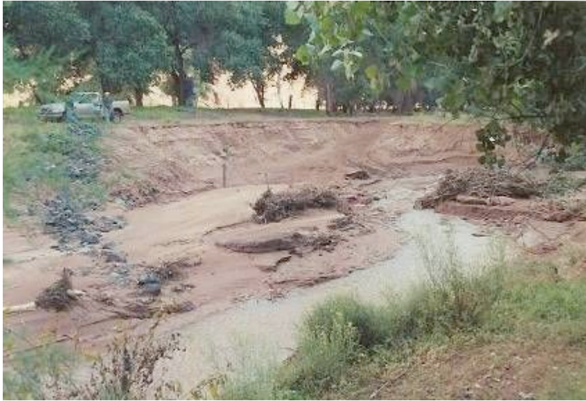
Road crossing with streambarb recently installed, Demo Site #6, Sept 1999.
