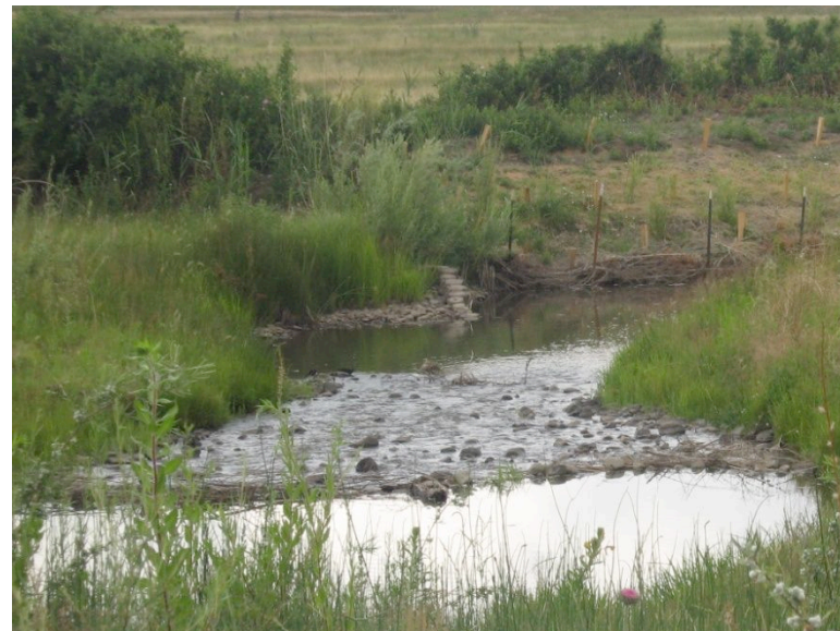
Wooden post vanes slow near shore velocities and capture sediment.
