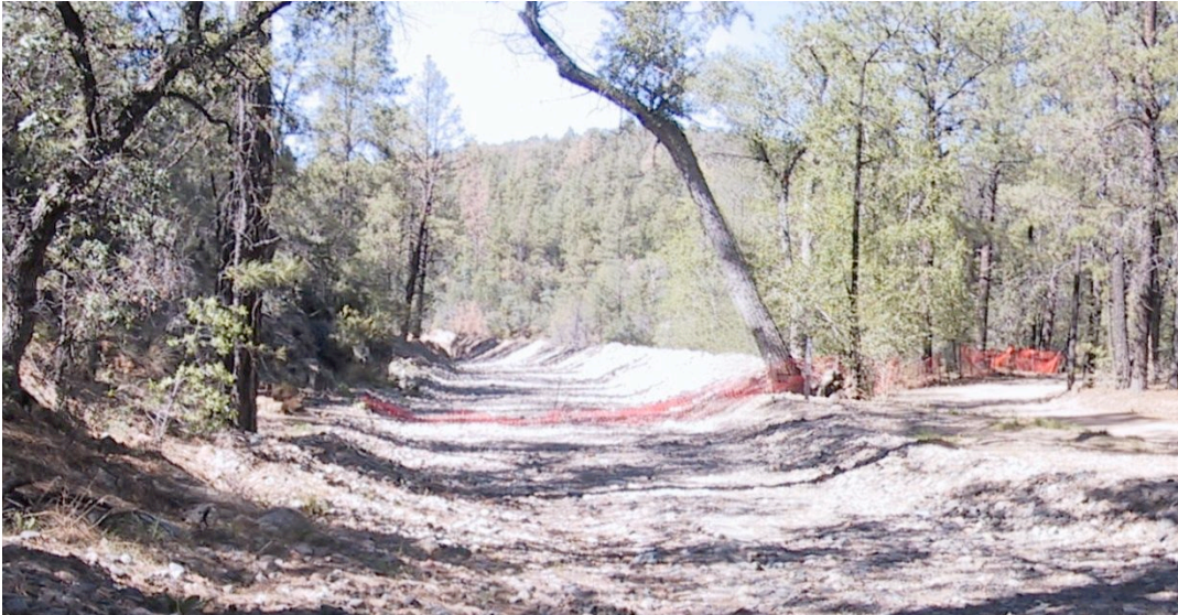
Looking downstream at upper end of project area. September 2003.
