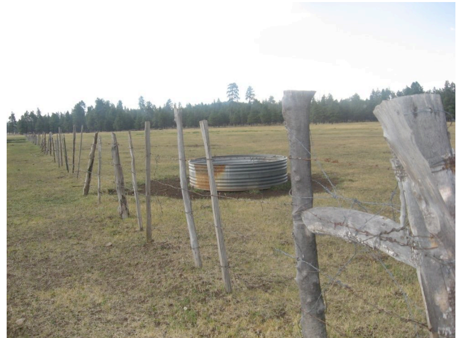
One of multiple drinkers and fence lines installed in the Gooseberry Creek Watershed.
