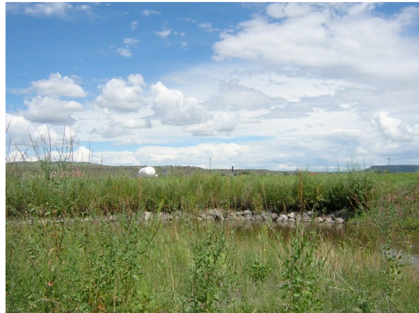
Same bank in 2006 after bank sloping, rock toe protection and re-vegetation.
