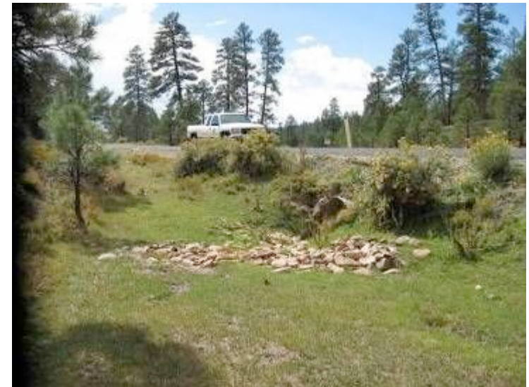
Rock inlet at culvert to hold grade, Demo Site #2, October 2007..
