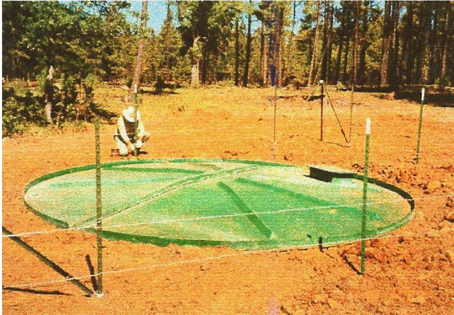
Rain catching storage tank just after completion of construction, before seeding. 2000.
