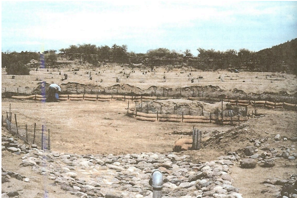
Building the backwater pond . July 2007.
