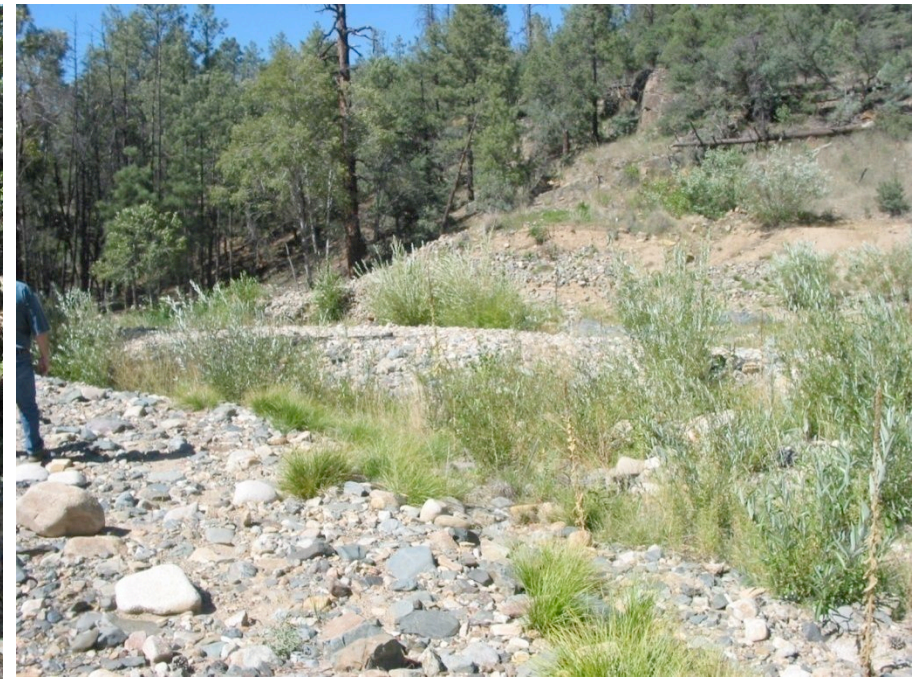
Restored channel looking downstream towards gabion location. September 2007.
