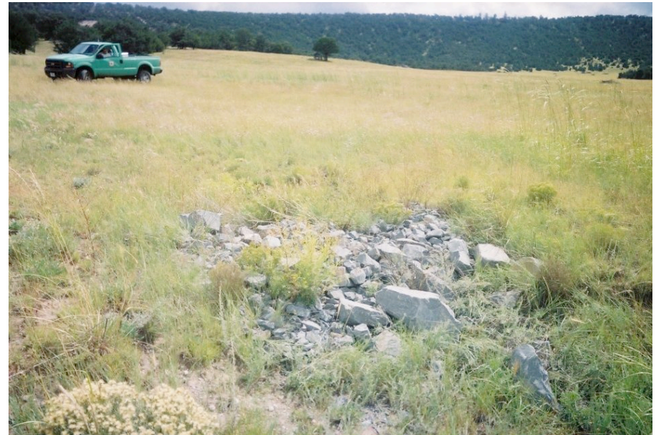
Repaired headcut becoming revegetated. September 2007.
