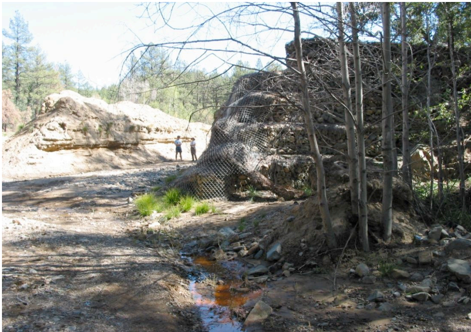
Gabion structure and accumulated sediment upstream. September 2003.
