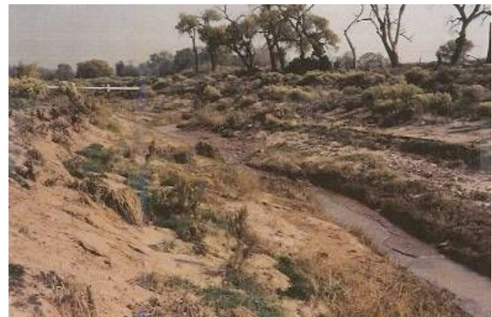
Photo showing channel adjustments. October 2003.
