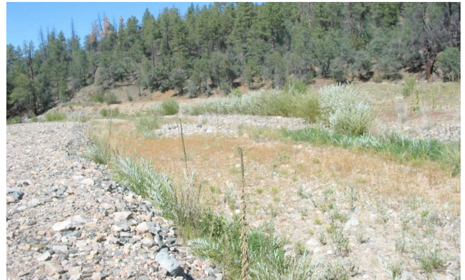
Restored stream channel upstream of removed gabion structure. September 2007.
