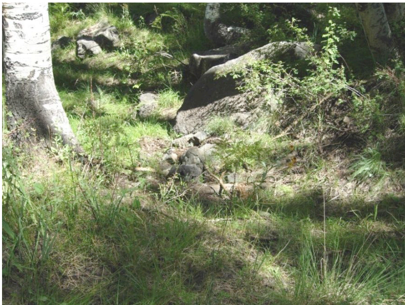
Recontoured channel where diversion dam was removed . 2007
