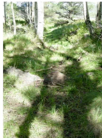
Diversion Dam removal and recontoured channel. 2007.
