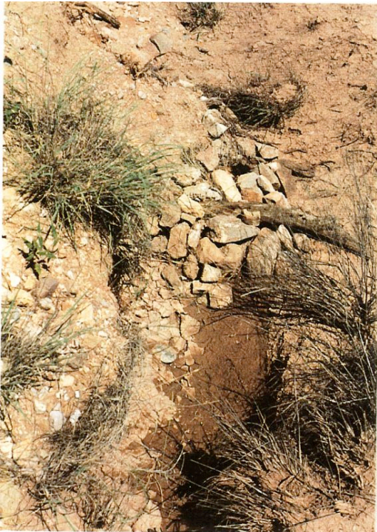
A small check dam structure as constructed in 1996
