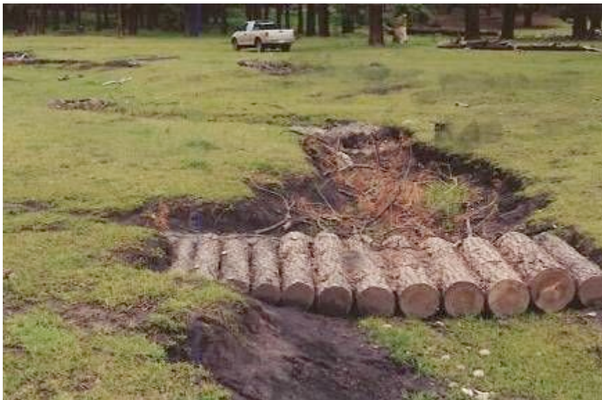
Log and sandbag structure with brush at Demo Site #4, June 2000.
