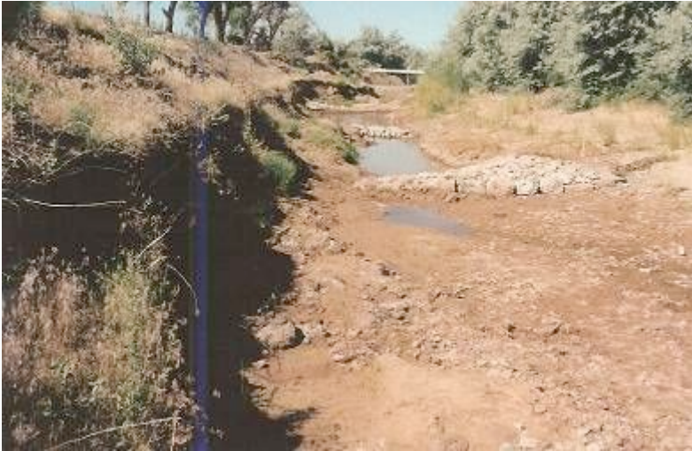
Rock baffle "induced meander" structures. July 1998.
