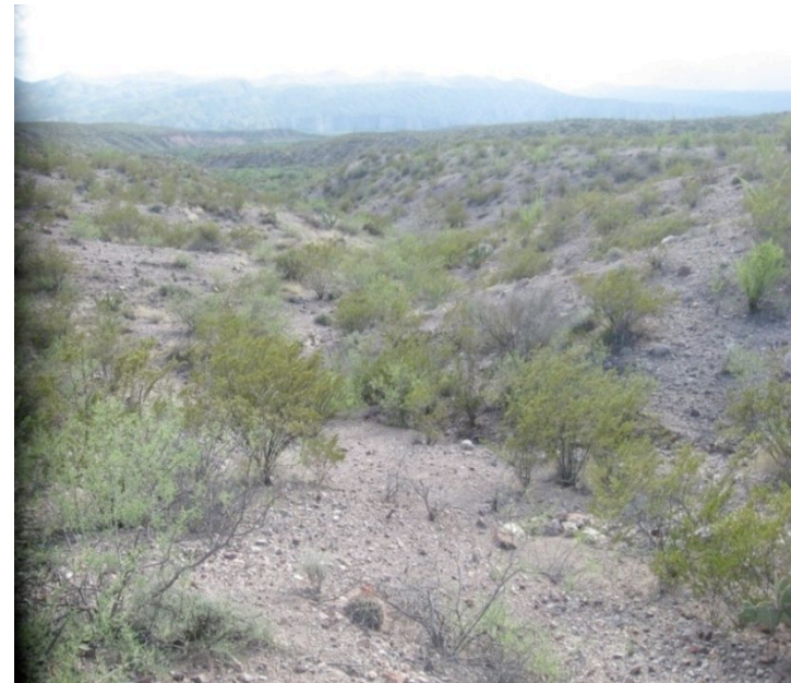
Overview of check dam structures in a tributary wash in Teran Watershed in 2007.
