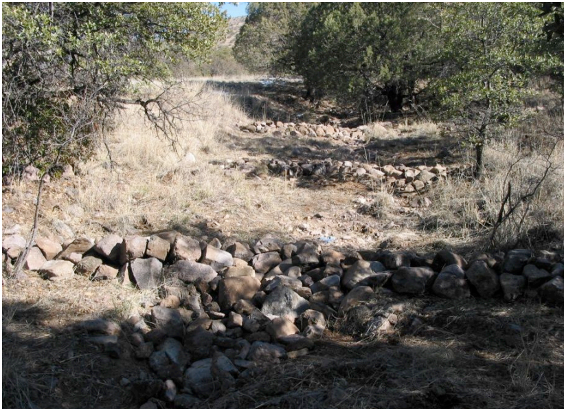
Structures were placed in series in even the smallest channels. 2004.
