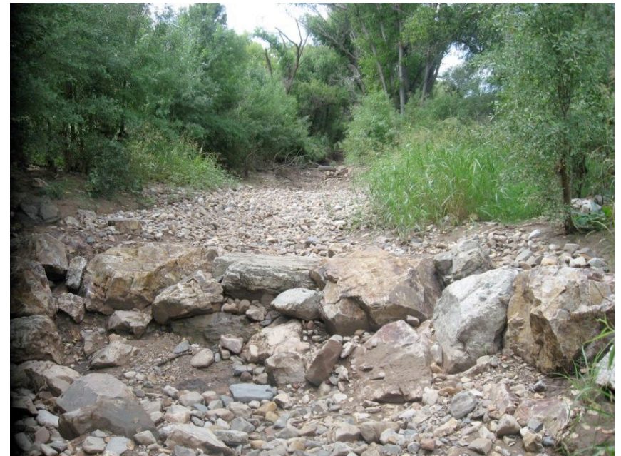
Upstream view of headcut remediation at Dike #3 removal site 2007.
