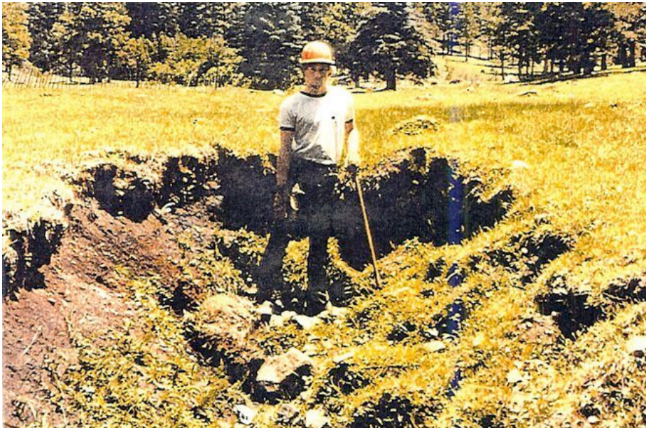
Pre-construction headcut. Summer 2000.
