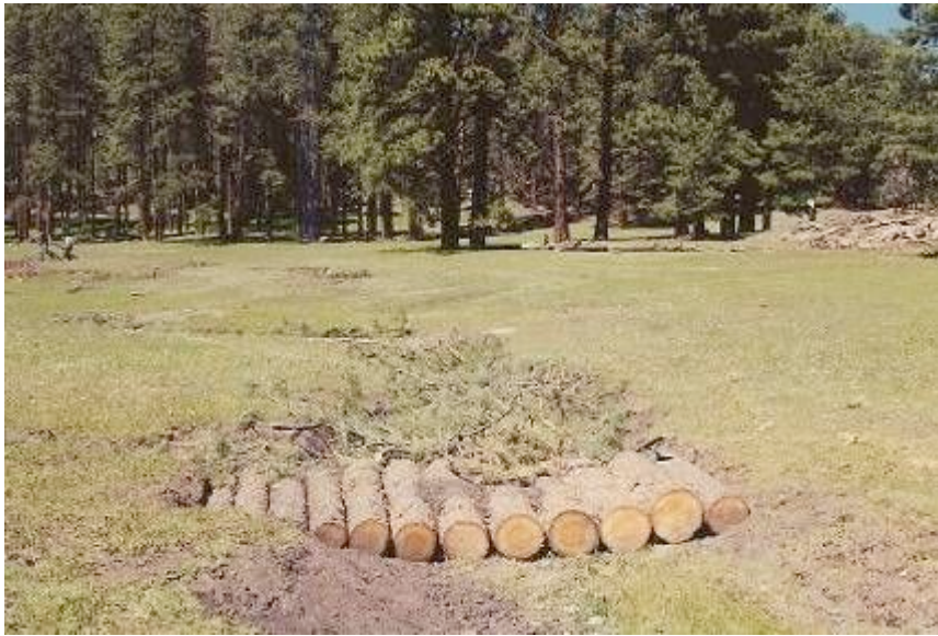
Log and sandbag structures at Demo Site #3, June 2000.
