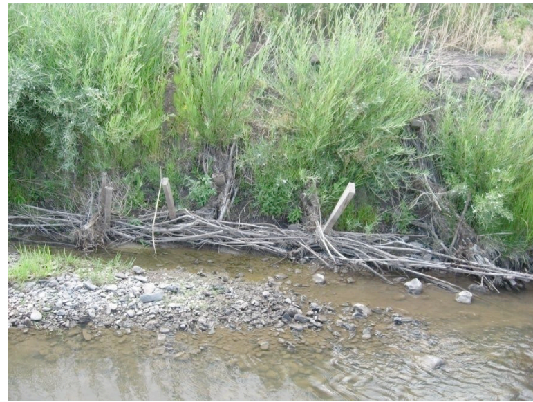
Willows sprouting from pole bundles. 2007.
