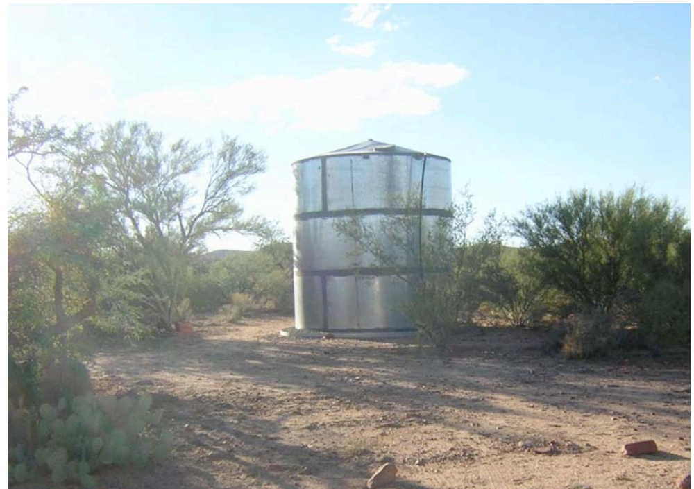
Pipeline and reservoir tanks were installed to distribute water from existing wells.
