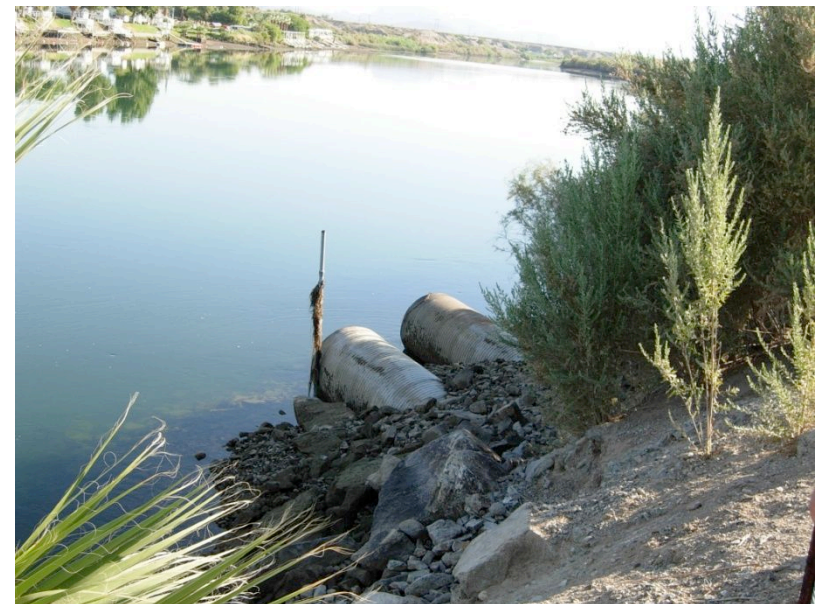
Water control structure, 2007.
