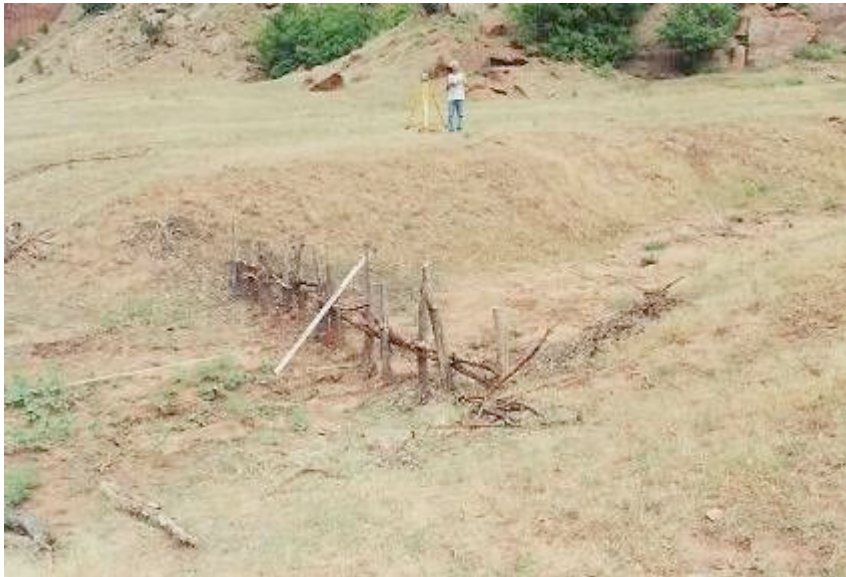
Erosion fence made from tamarisk posts, Demo Site #5, June 1999.
