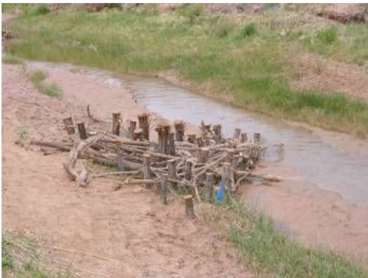
Post baffle structure. May 2003.
