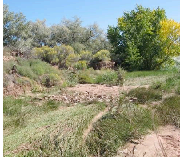
Rock, post, rock baffle structure. October 2007.
