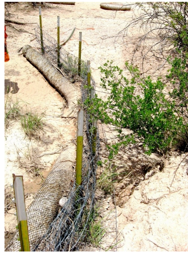
V-mesh spreaders/T-Bar sediment traps. Scour on the downstream side exists. Waddles were added later to mitigate scour and downcutting. July 2007.
