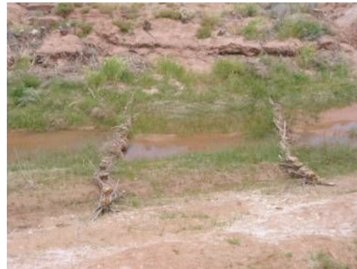
Post and single-rock riffle structure. May 2003.
