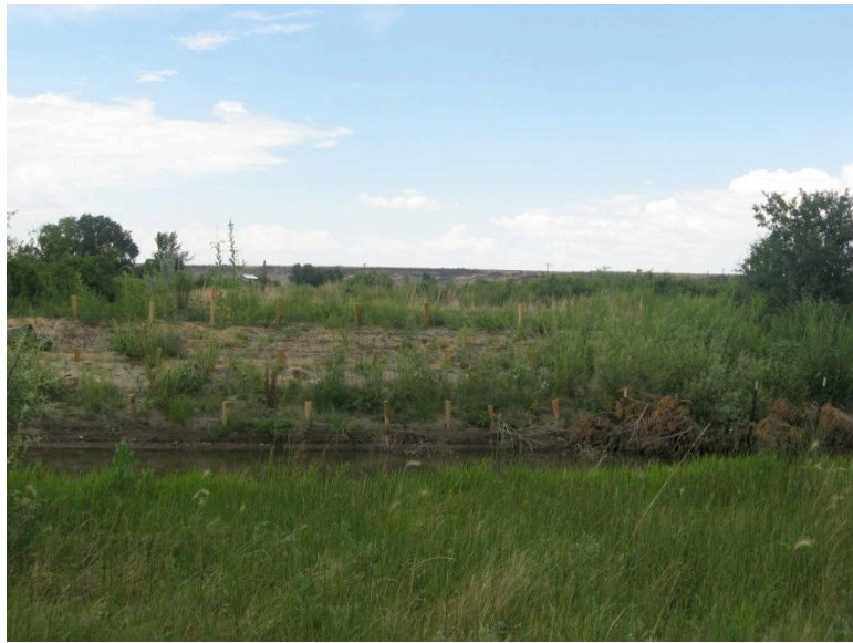
Bank re-sloping with re-vegetation. 2007
