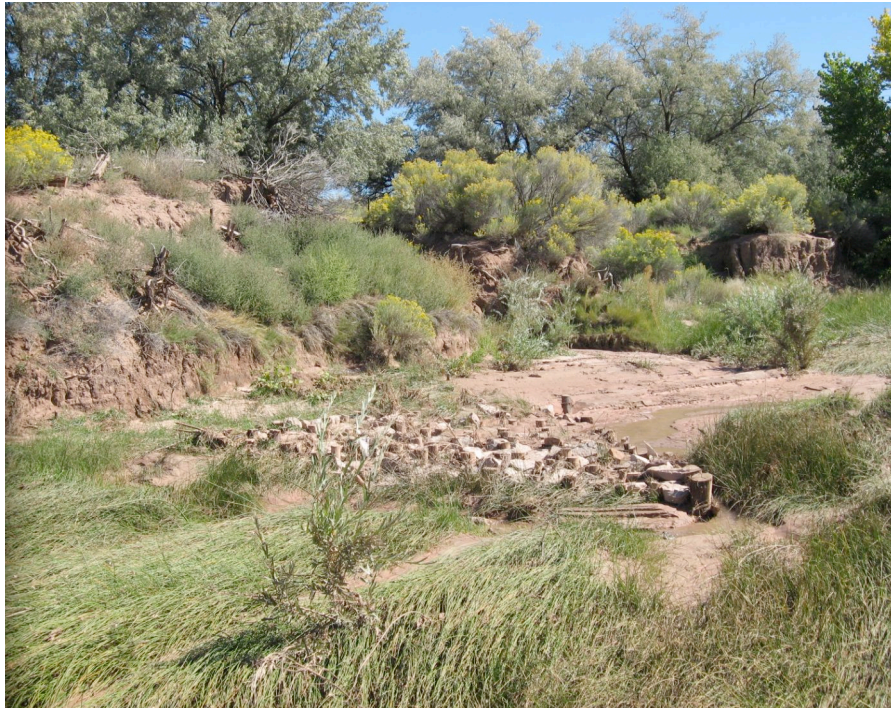
Figure 20. Induced meander structure, or baffle, at the Hubbell Trading Post project site (#00-104WPF).
