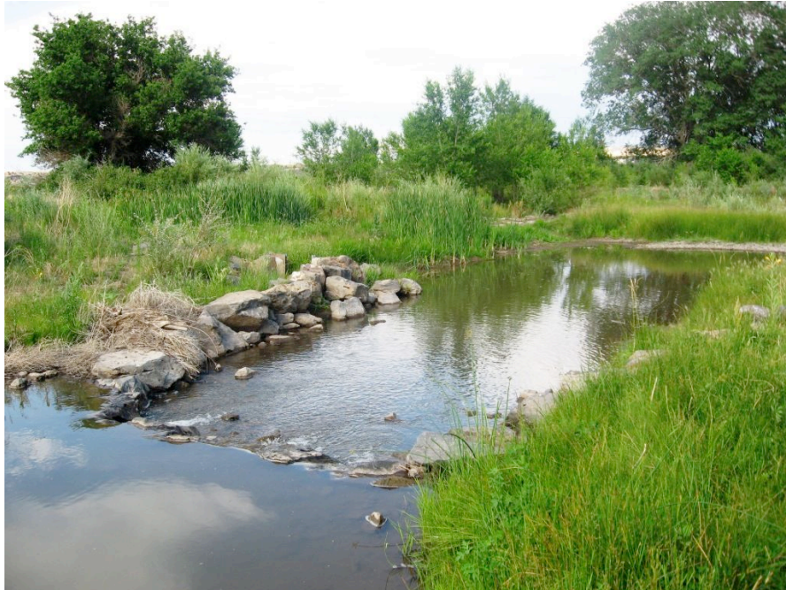
Figure 16. Cross-vane weir structure demonstrates improved diversion at the LCR Demo project site (#99-092WPF).
