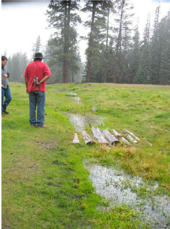
Figure 15. Log and sand bag structure at the Tsaile Creek Watershed Restoration Demonstration project (#96-0025WPF).
