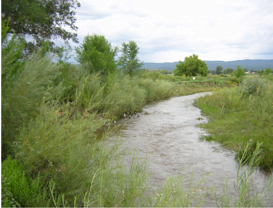
Figure 10. Vertical willow bundles used for bank stabilization at the Little Colorado River Enhancement Demonstration Project (#99-092WPF).
