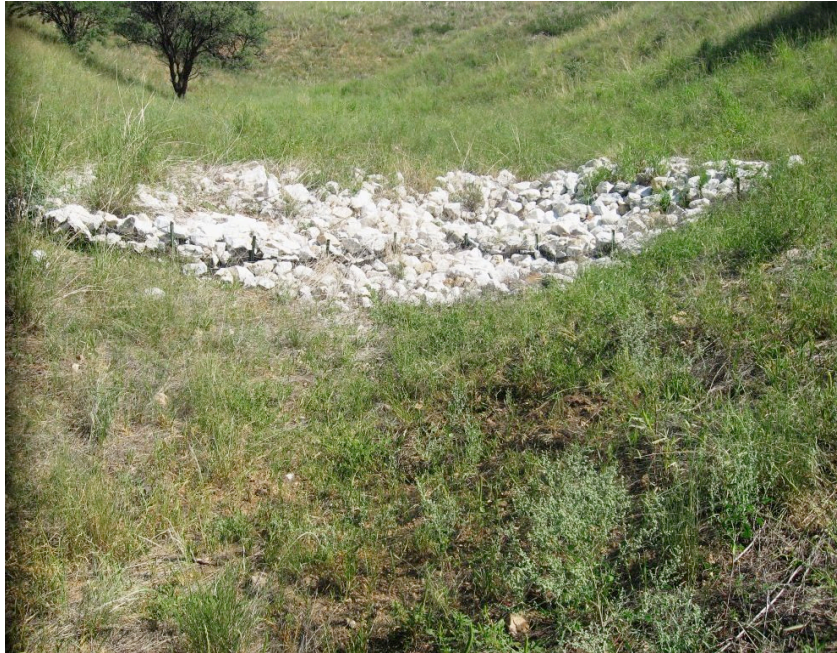
Figure 14. Rock structures stabilize headcuts at Oak Tree project (#97-034WPF).
