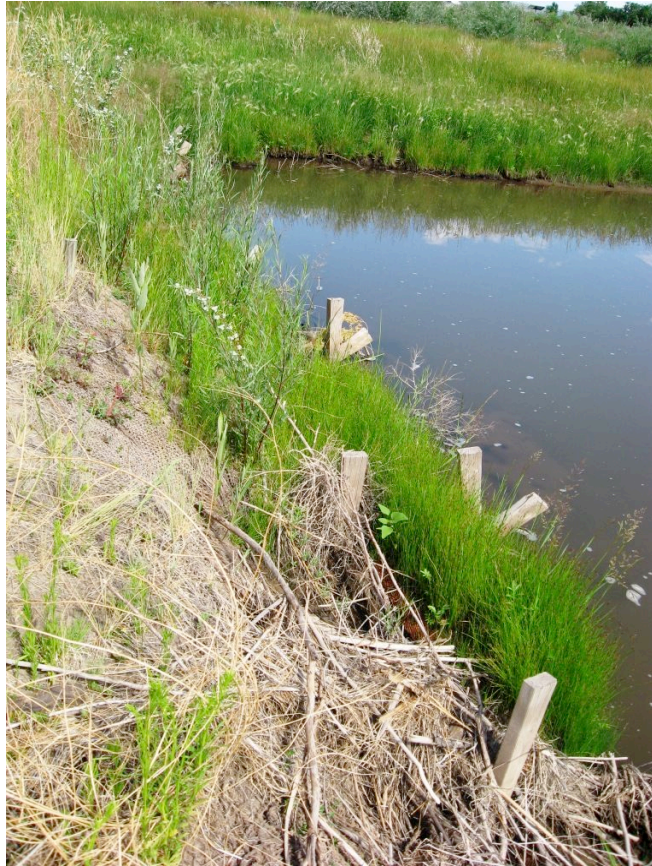
Figure 12. Bio-logs provide temporary bank protection along the Little Colorado River (#99-092WPF).
