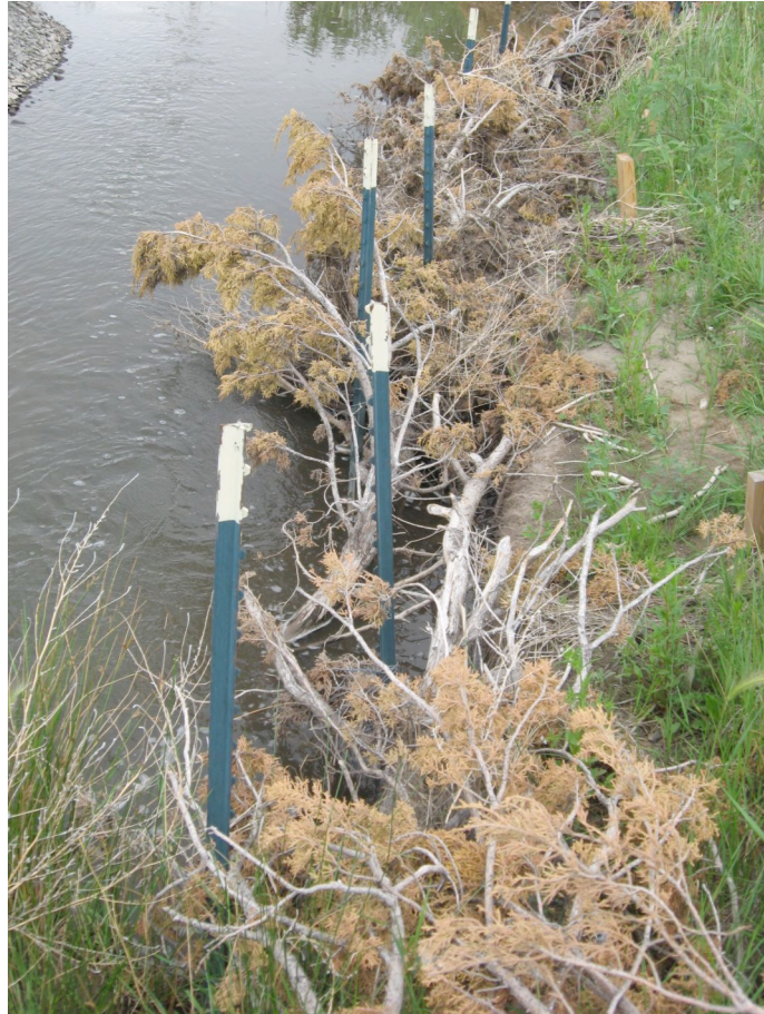
Figure 11. Brush revetments on the Little Colorado River (#99-092WPF).
