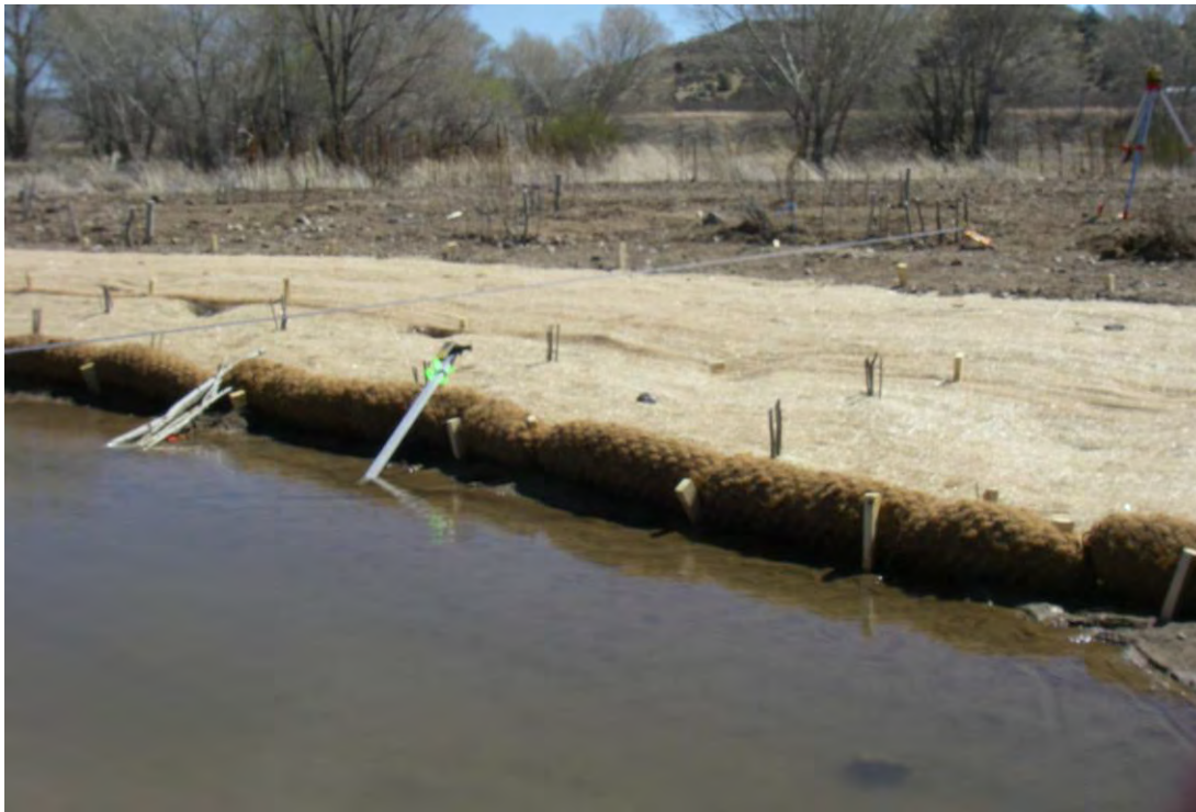
Figure B 30: BEHI 6 bank profile post-construction April 2009.
