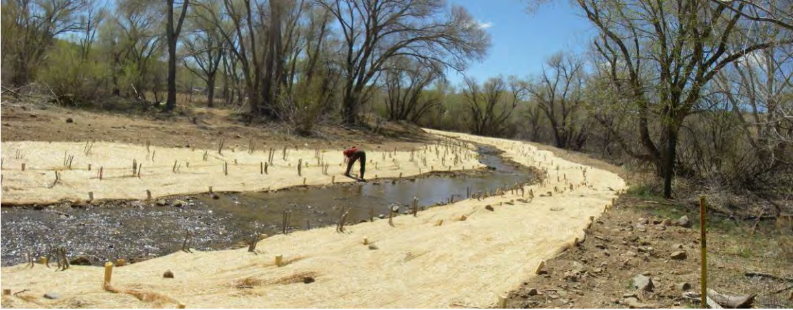
Figure C 11: Upstream from PP-2, Reach 1 taken April 2009.
