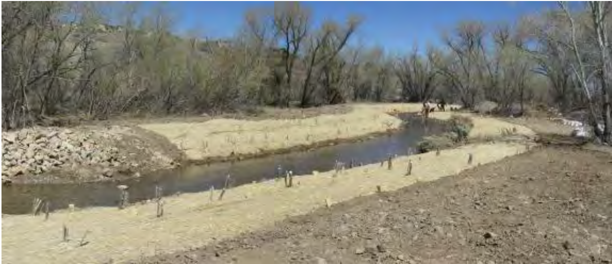
Figure C 6: Downstream from PP-1, Reach 1, taken April 2009.
