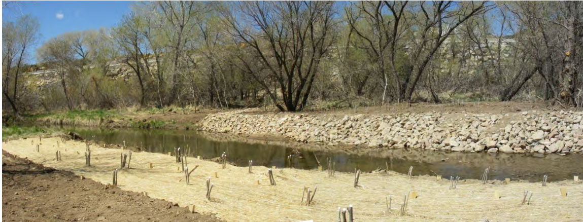
Figure C 1: Upstream from PP-1, Reach 1 taken April 2009.
