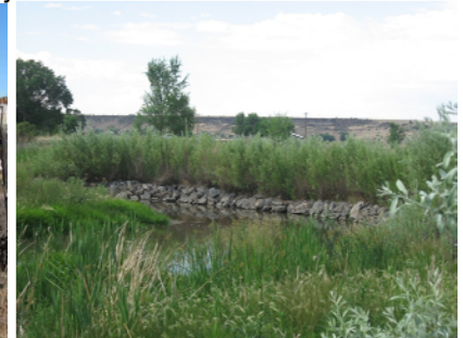
Initial construction and final product for one eroding bank on the LCR Demo Project
