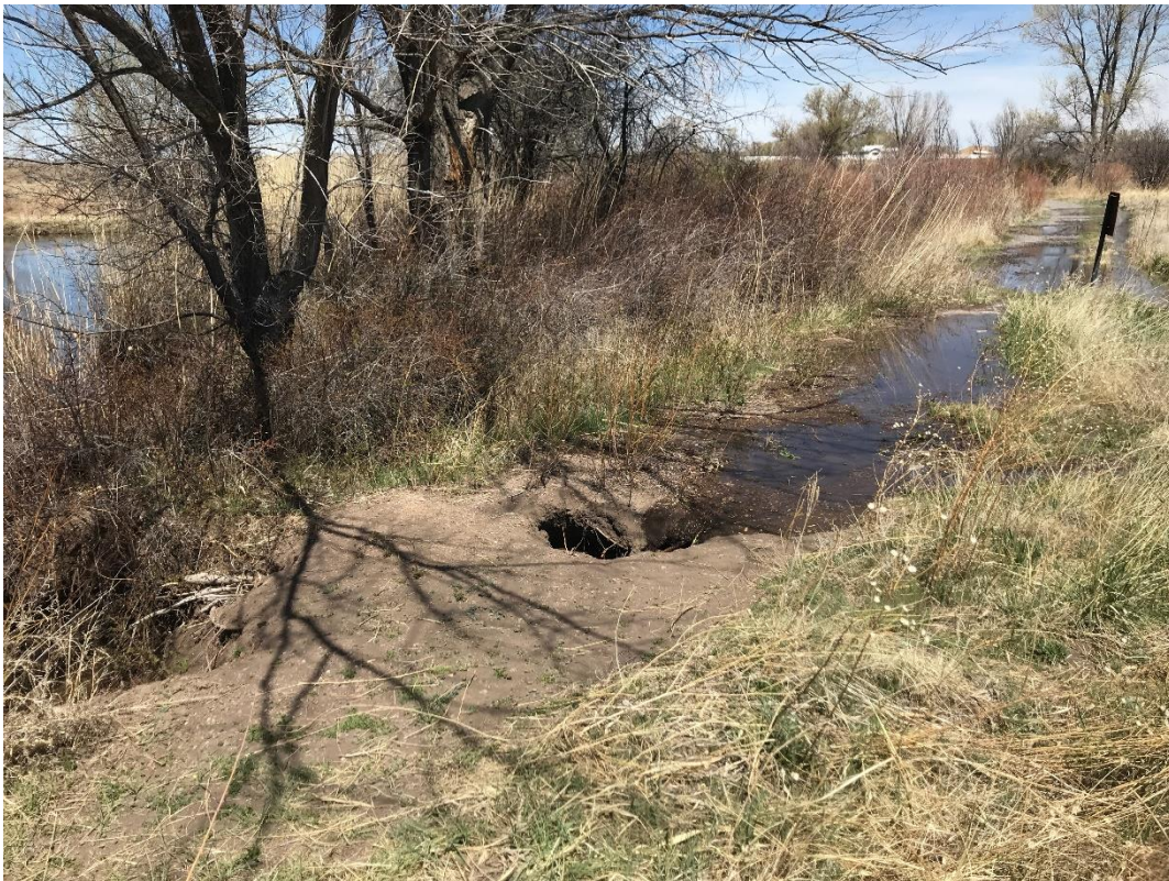
Figure 8: River Walk trail with erosion from nearby river cutbank exacerbated by agricultural tailwater.
