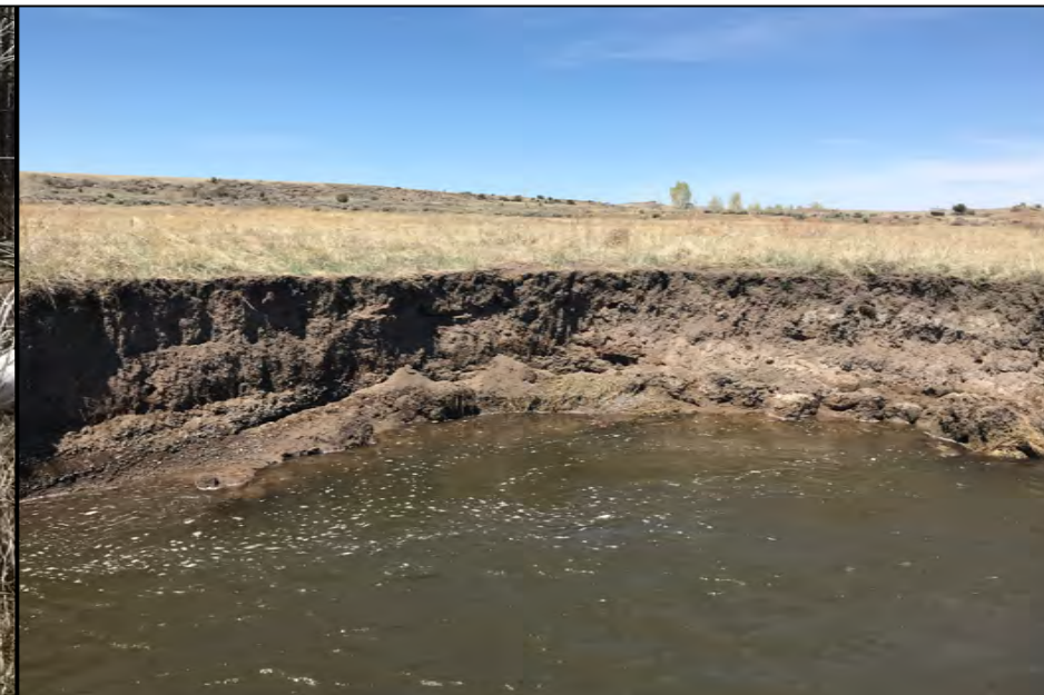
D Beaver Dam Breach at Irrigation Point of Diversion
