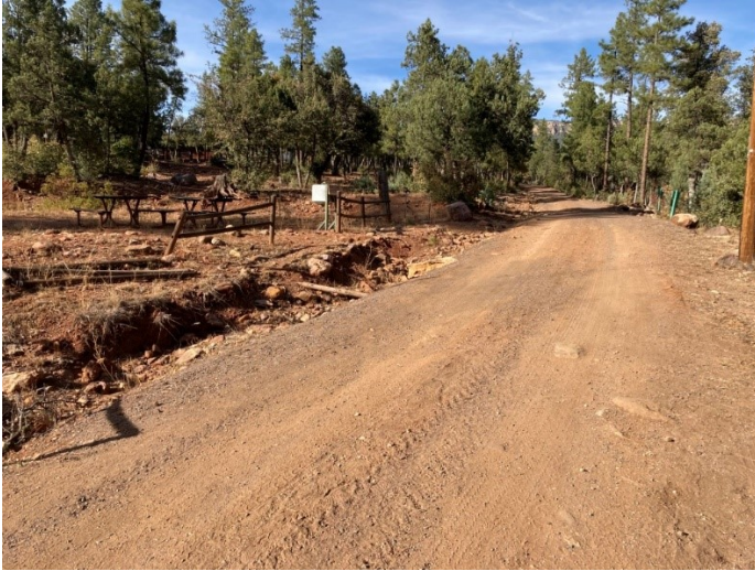
Figure 3. Existing road drainage
