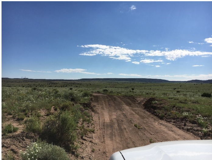
Figure 4. Rolling dip installed on dirt road in Apache County
