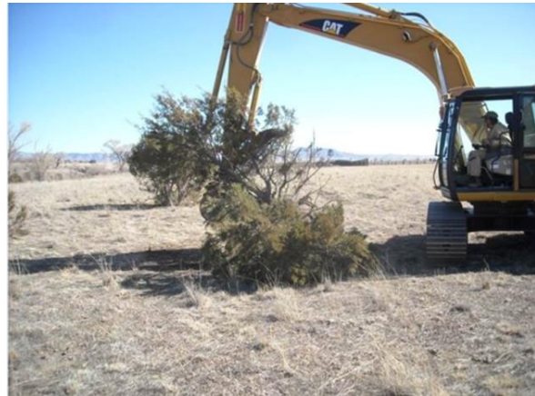
Cat 308 excavator with thumb
