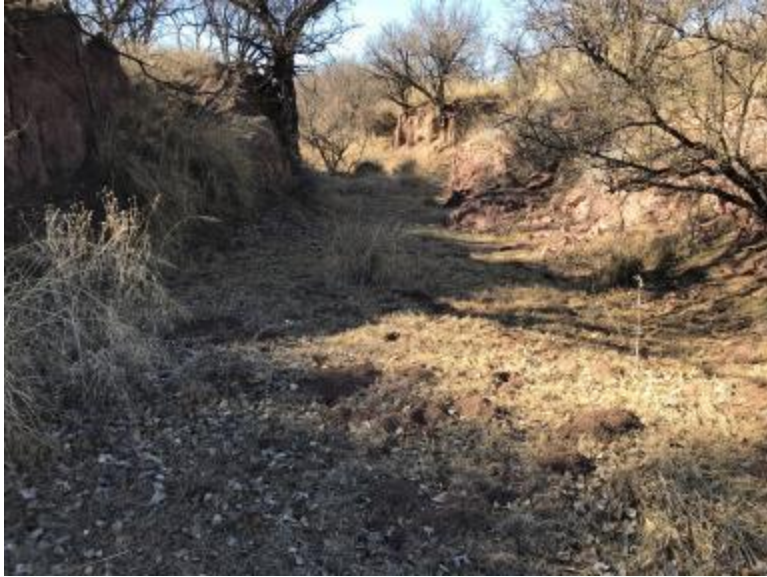
Looking upstream at incised tributary caused by railroad (GPS point 25): Flows from the respective culvert contributed to downcutting resulting in this massive headcut.
