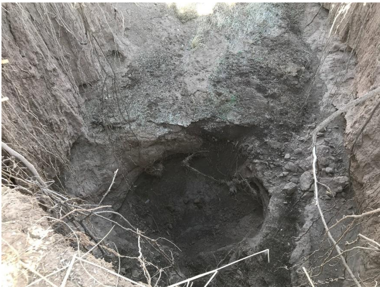
Figure 3a: Looking down at plunge pool of a major active headcut (vicinity of GPS point 9)
