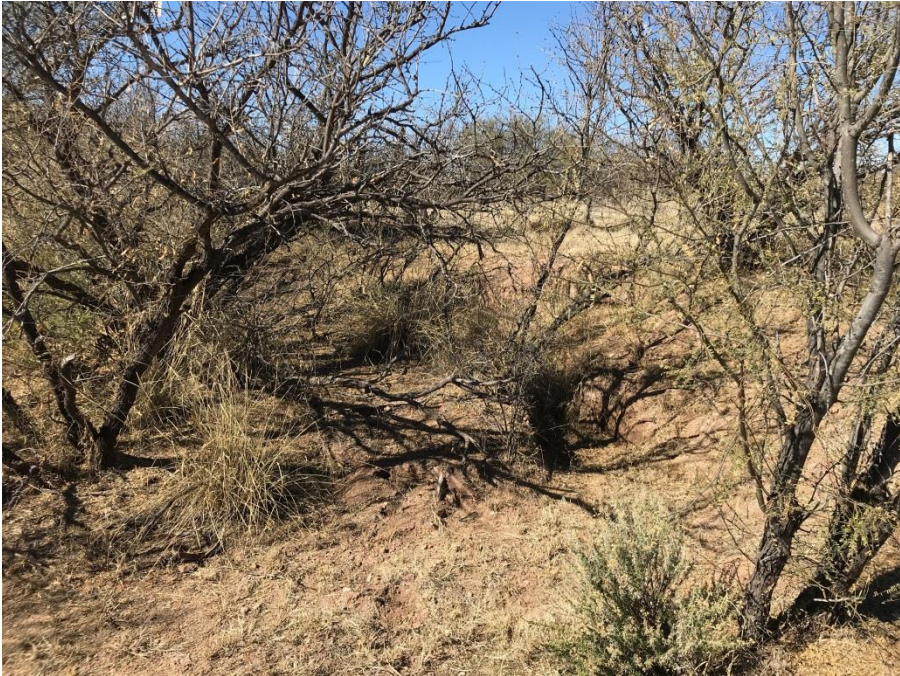
Erosion of the down-valley side of the berm for the mentioned dirt tank
