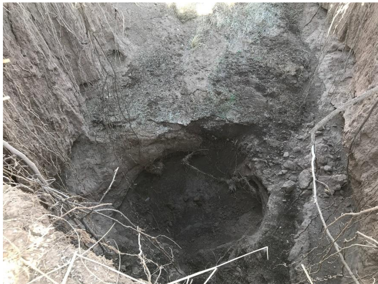
Figure 7: Looking down at plunge pool of a major active headcut (vicinity of GPS point 9)
