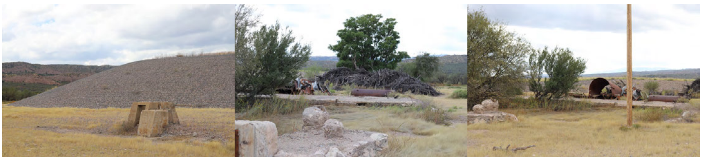
Capped Mine Tailings and Abandoned Mill Equipment at Klondyke Tailing Superfund/WQARF Site
