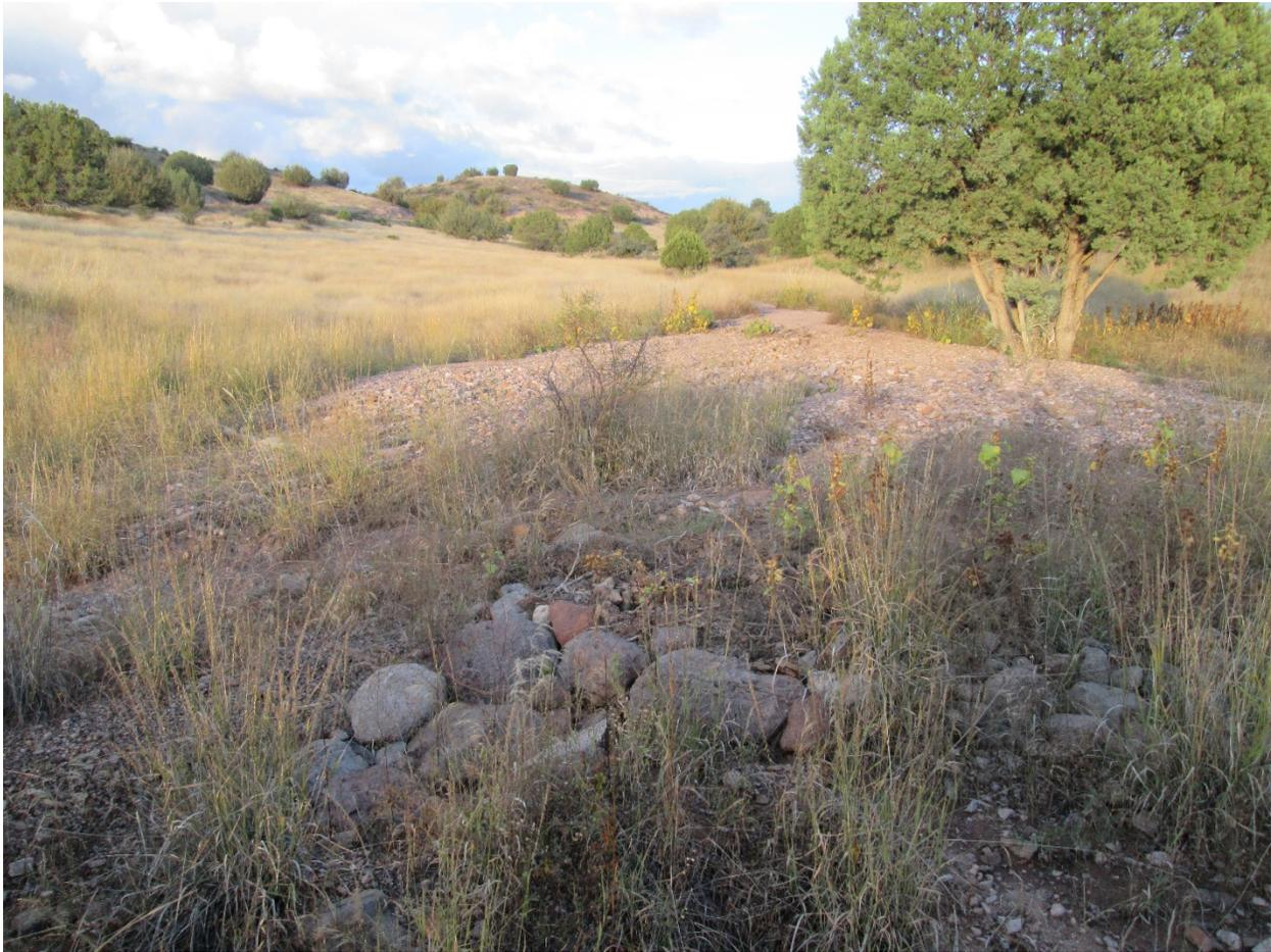
**An** overall view showing the October 2012 site 2+ years later. The initial deep channelization has been entirely covered and several small media lunas in the foreground are spreading any remaining flows across the lower portion of the site. As additional sediment is collected at this location, vegetation and ground cover should continue increasing.
