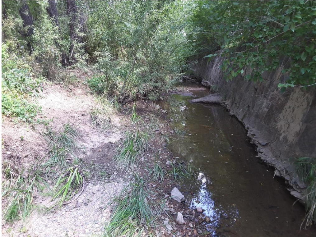
Figure 7. Retaining wall with scour occurring along toe.
