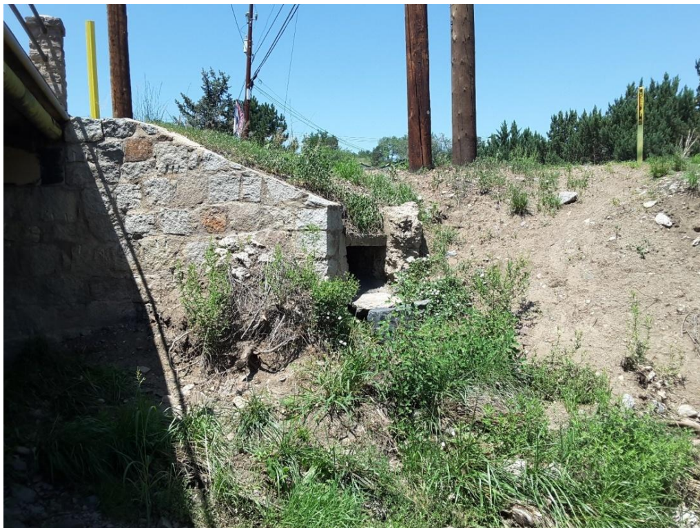
Figure 3. Stormwater outlet and bank erosion.
