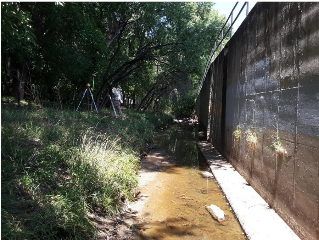
Figure 2. Retaining wall encroachment into the active channel.
