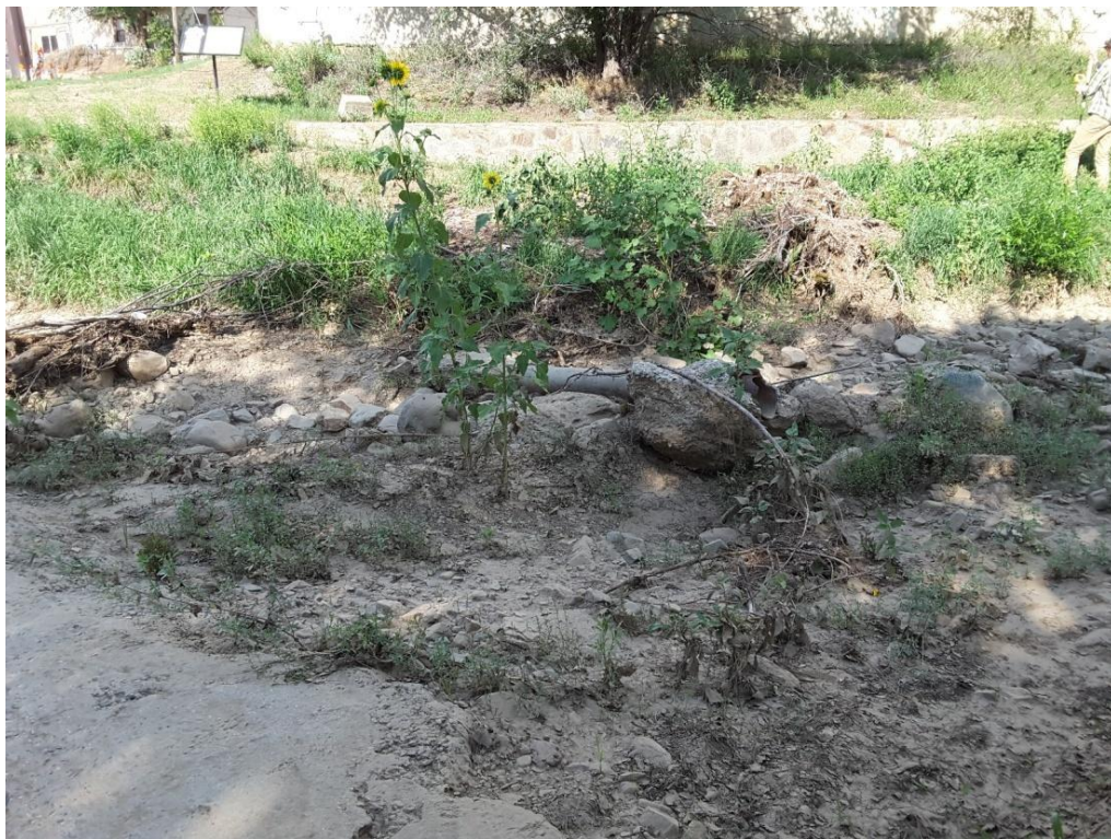
Figure 10. Abandoned sewer line in channel.
