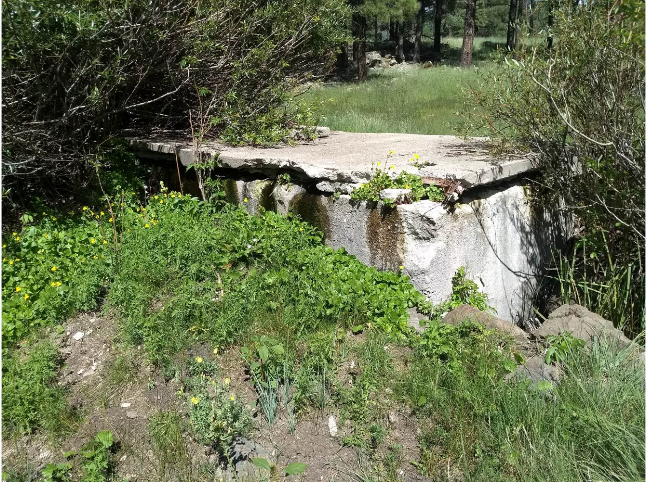
Figure 1. Abandoned concrete springbox slated for demolition.
