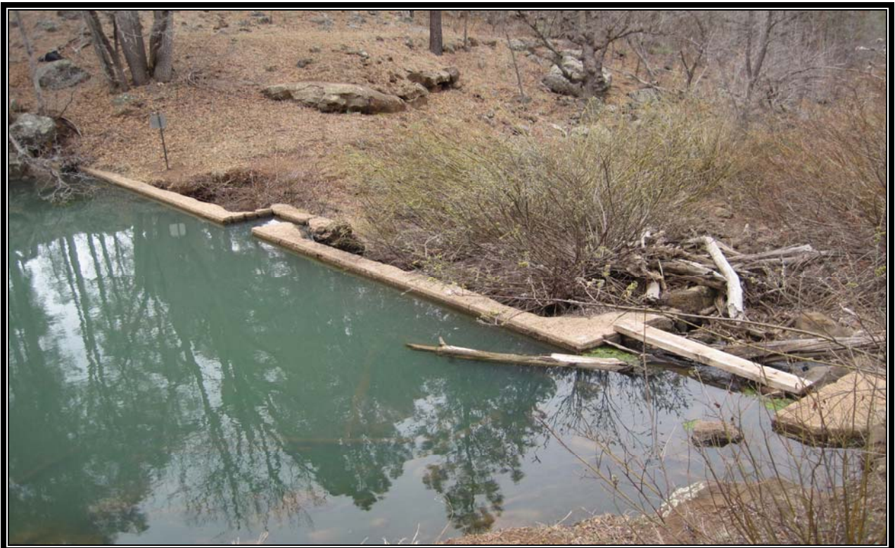
Figure 23. AZ Q:13:27 (ASM), Feature 4, looking west showing the vertical upstream face, the center outlet, and the northeast spillway.
