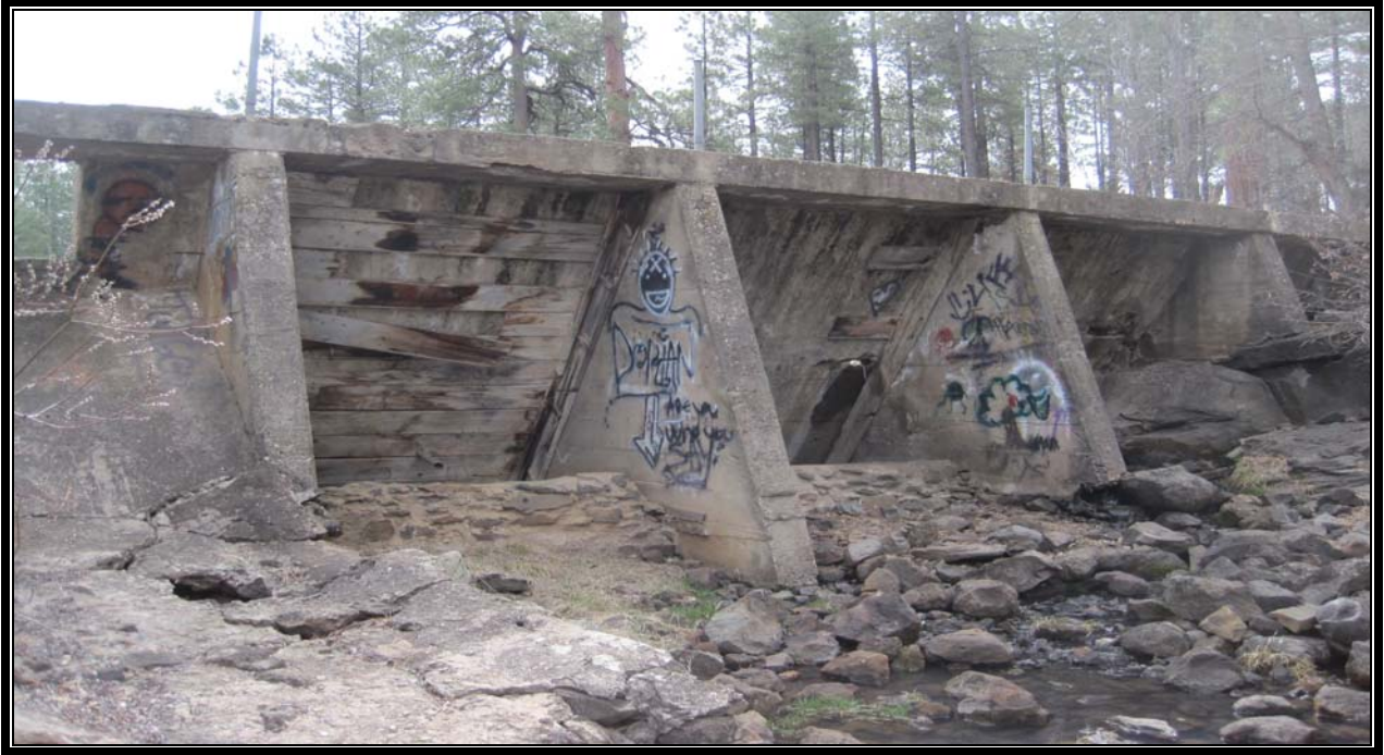
Figure 18. AZ Q:13:27 (ASM), Feature 4, looking southeast at the buttresses on the downstream (northwest) face of the dam.
