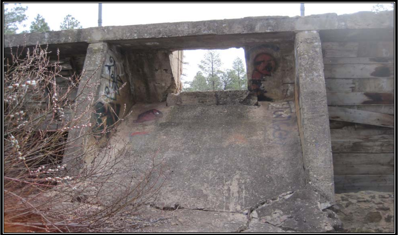
Figure 20. AZ Q:13:27 (ASM), Feature 4, looking southeast at the spillway near the center of the downstream (northwest) face of the dam.
